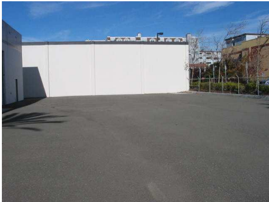
Photo 2. View looking north of rear parking area.
