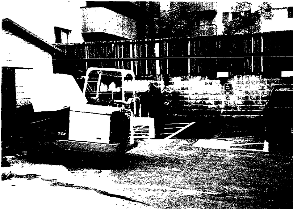
Photo looking east of the excavation area. The asphalt has been installed. Note the handicap parking space and sign.
