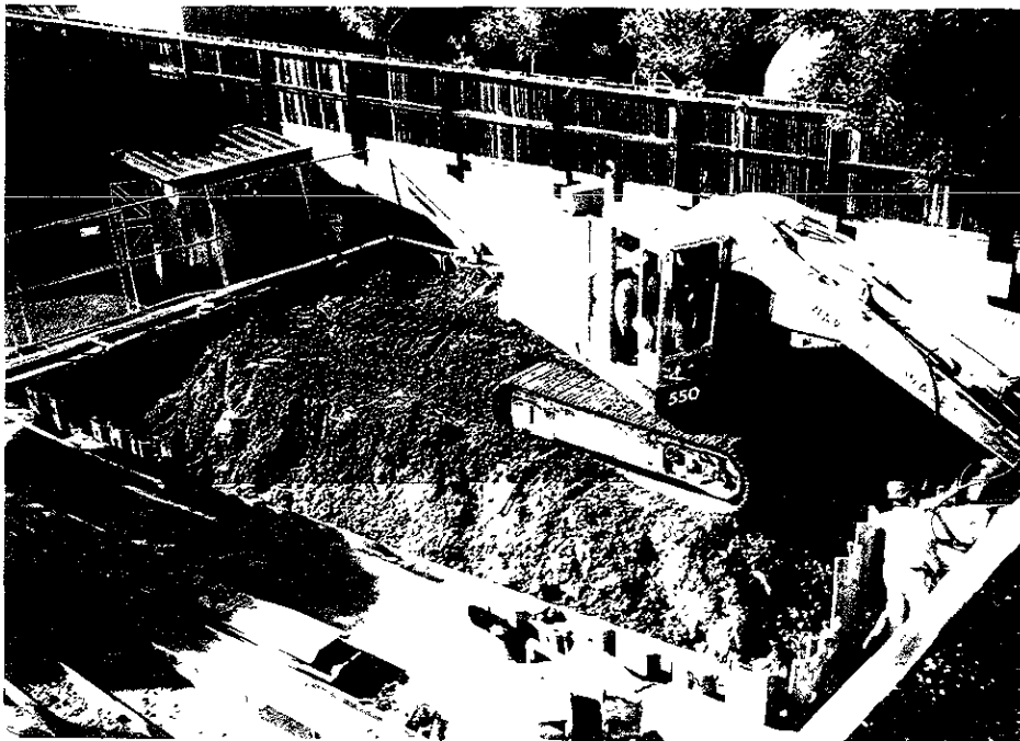
Photo of nearly-completed shoring installation
