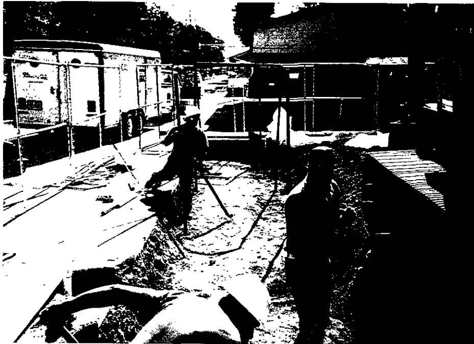
Photo looking south of the eastern portion of excavation area showing the top of the concrete-encased utility trench. Workers building a containment structure.
