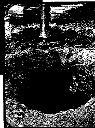
Drilling of large diameter shafts - Photo at right shows two shafts drilled within close proximity to each other which caused the collapse of the sidewall of one shaft into the other shaft.
