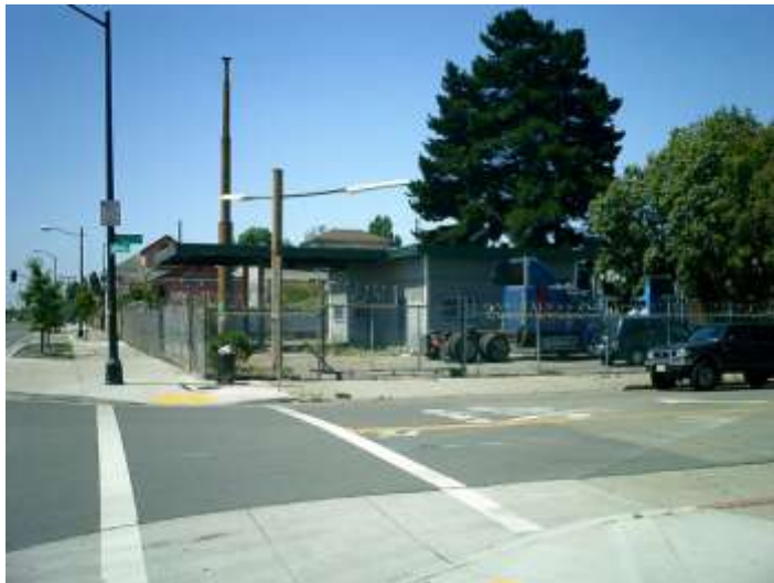
Photograph No. 1 - view southward of subject property from corner of Mandela Parkway and 13 th Street. Office building and fenced lot used for truck power unit storage. Fuel dispenser canopy on left side of building at former fuel dispenser locations.
