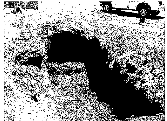
Photograph 4 shows the area excavated at OP-2 (6 feet in depth).
