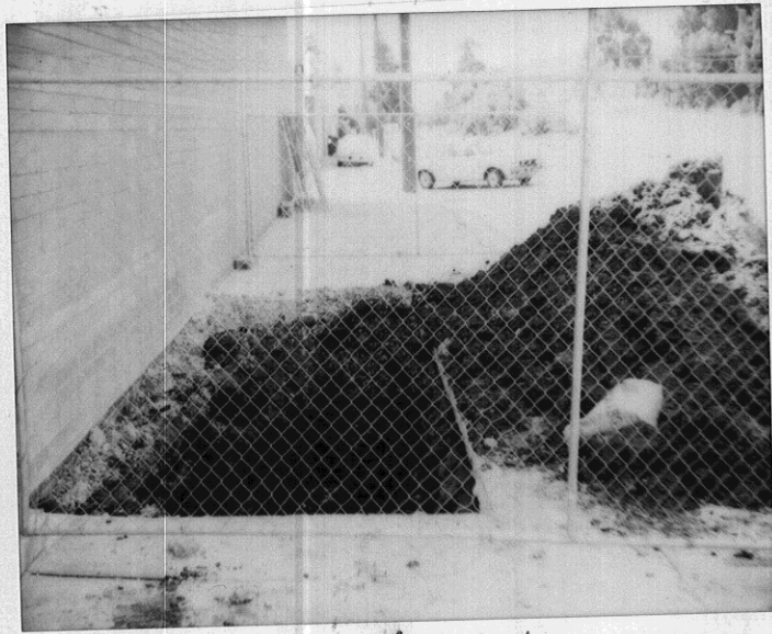
5/11/92 Sandi Metal Works 976 23rd - 500 gal gas pit
