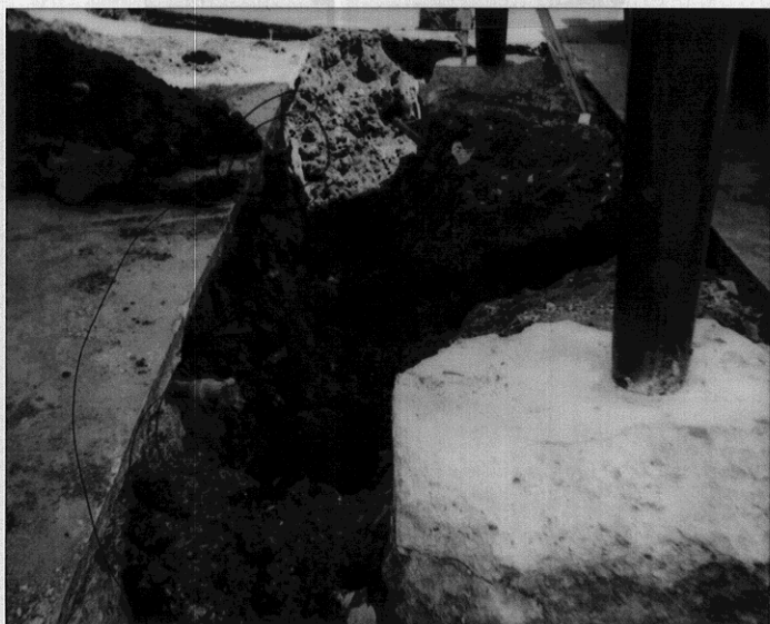
Unidentified piping. Probably from former gas station →
