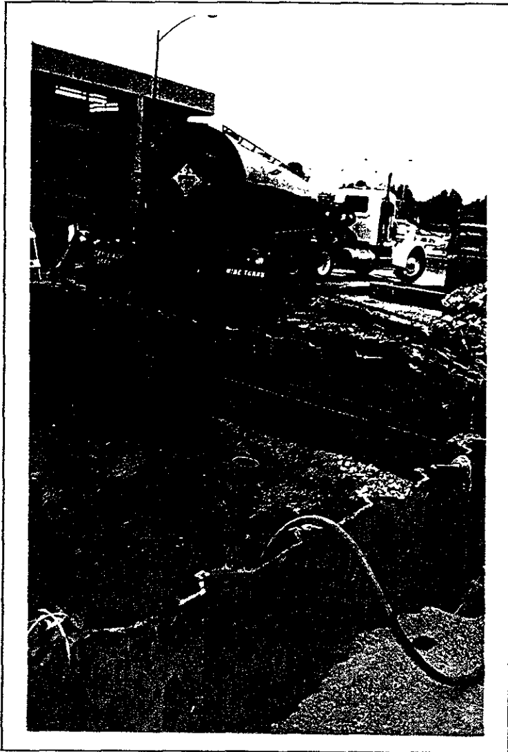
Photo E : H&H pump truck vacuuming the 10,000-gallon UST.
