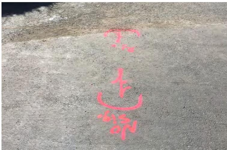
The photo to the left shows the “unknown” finding that was marked on the asphalt patch on site. This unknown finding was approximately 2’ in depth.
