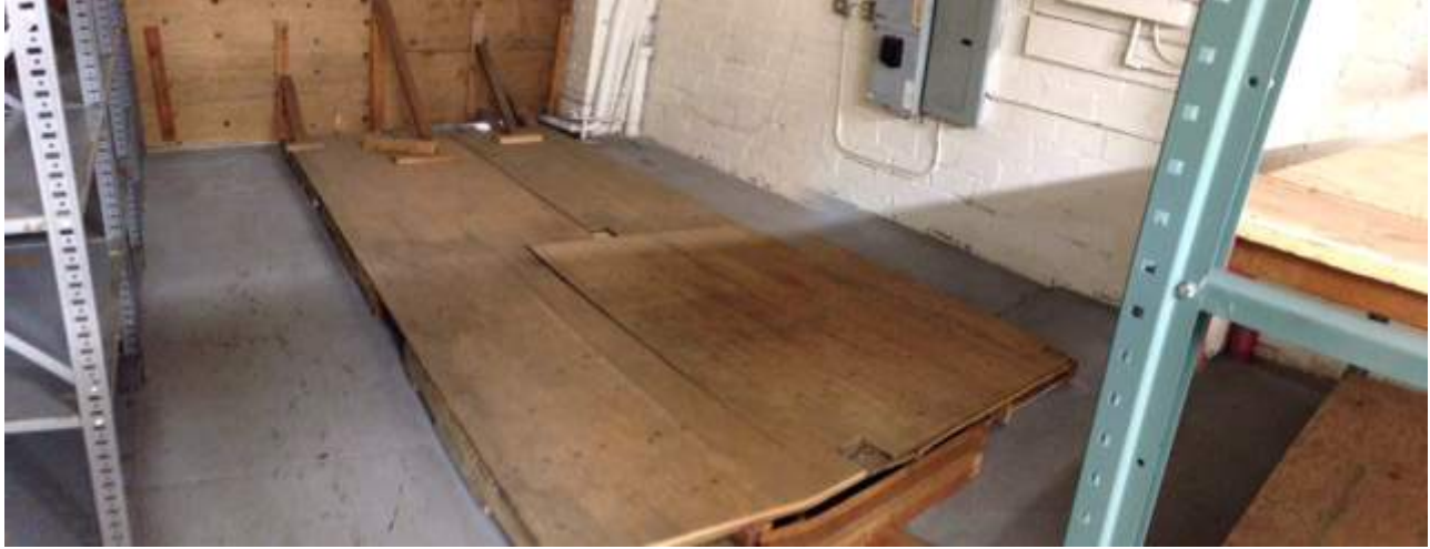
Photo 11: Subject Site (Facing Southwest) 3820 Penniman Avenue Interior Storage Warehouse - Floor
