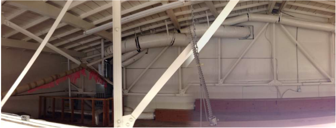
Photo 29: Subject Site (Facing Southwest) 3820 Penniman Avenue Interior Mezzanine Storage Area
