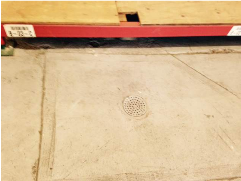
Photo 25: Subject Site (Facing Southeast) 3820 Penniman Avenue Interior Storage Warehouse - Drain
