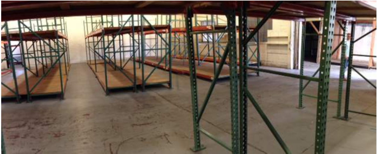
Photo 14: Subject Site (Facing East) 3820 Penniman Avenue Interior Storage Warehouse
