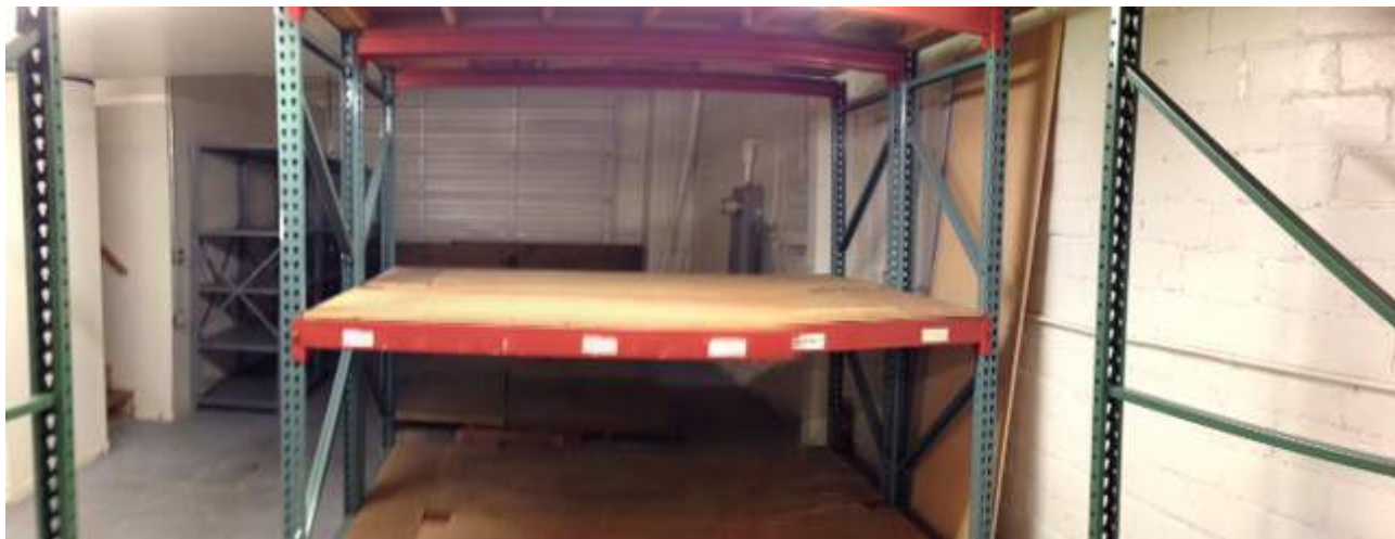
Photo 9: Subject Site (Facing Southwest) 3820 Penniman Avenue Interior Storage Warehouse - Racks, Roll Up Door
