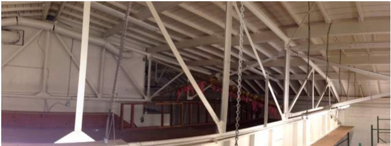
Photo 30: Subject Site (Facing West) 3820 Penniman Avenue Interior Mezzanine Storage Area
