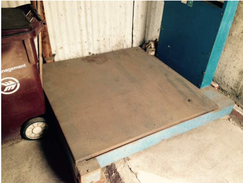
Photo 21: Subject Site (Facing North) 3820 Penniman Avenue Exterior Associated Paved area and Storage Shed - Scale
