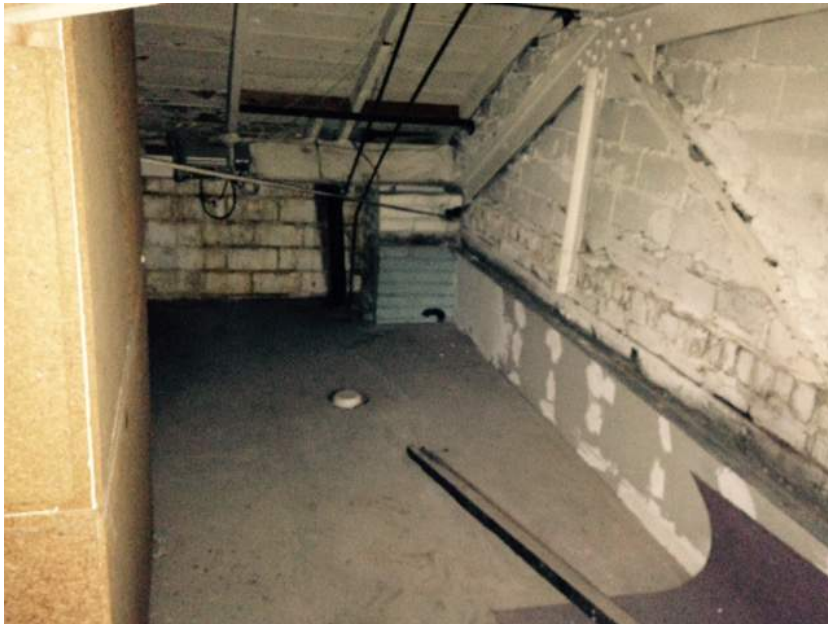
Photo 26: Subject Site (Facing Northeast) 3820 Penniman Avenue Interior Mezzanine Office Area
