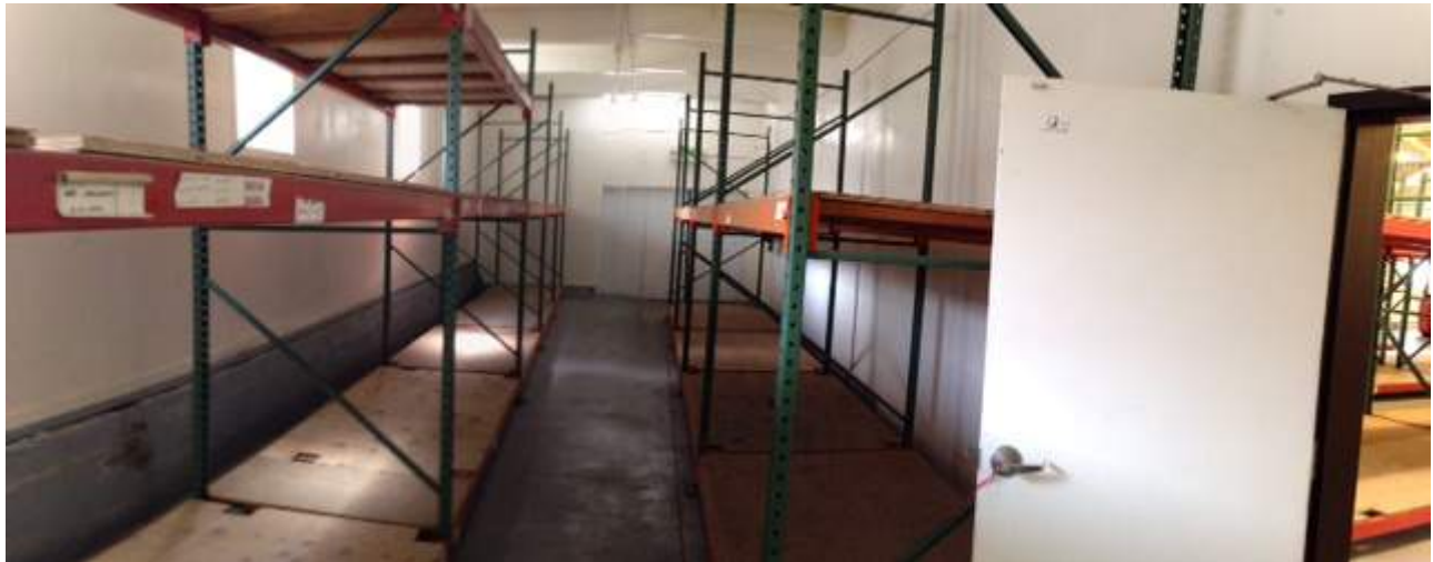
Photo 16: Subject Site (Facing Southeast) 3820 Penniman Avenue Interior Storage Warehouse
