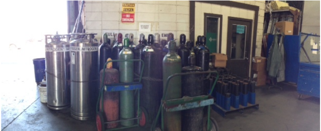
Photo 11: Subject Site (Facing North) Mechanical Warehouse - Compressed Gas Storage
