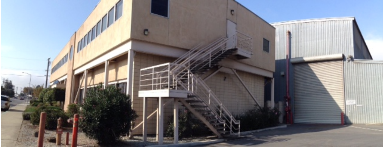
Photo 1: Subject Site (Facing Southwest) Partial Two-Story Commercial Office/Warehouse Building
