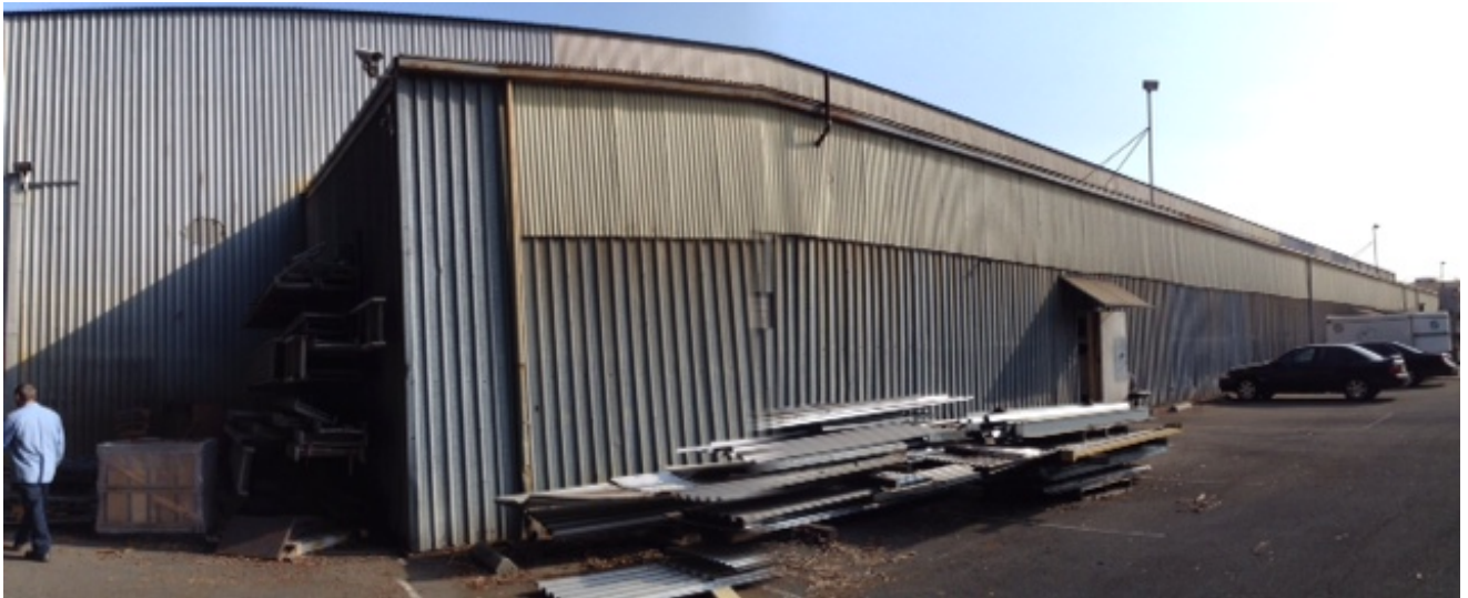
Photo 2: Subject Site (Facing Northeast) Partial Two-Story Commercial Office/Warehouse Building
