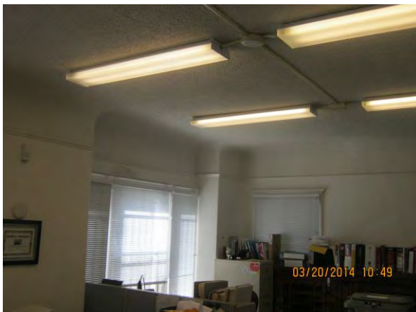
Interior view 5203 Dover Street building
