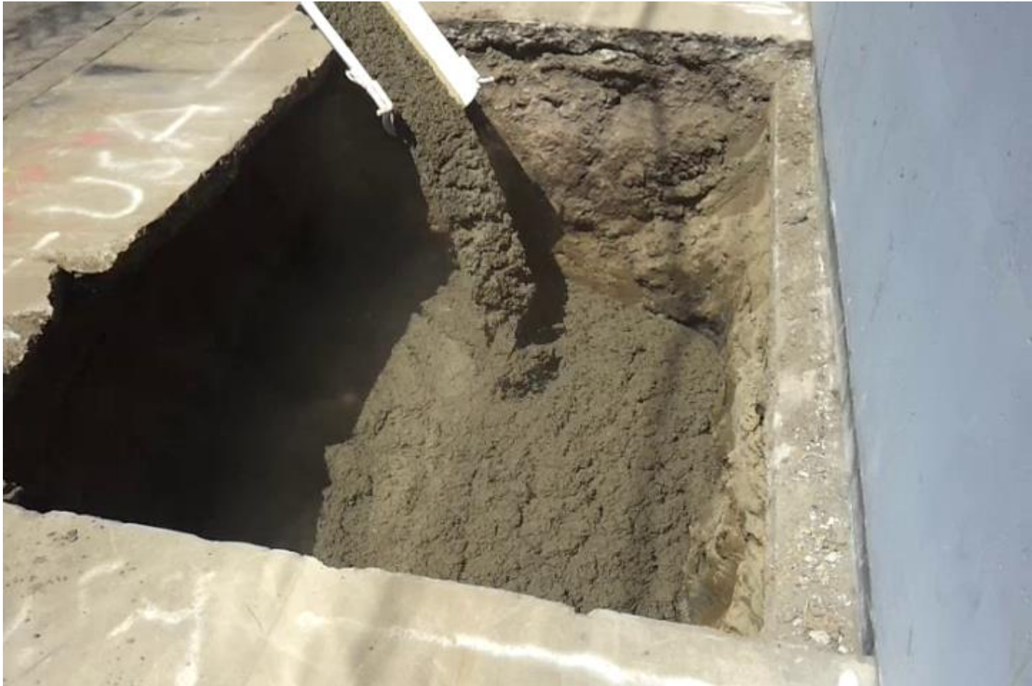
Photo 7: Excavation being backfilled with self-compacting fill.
