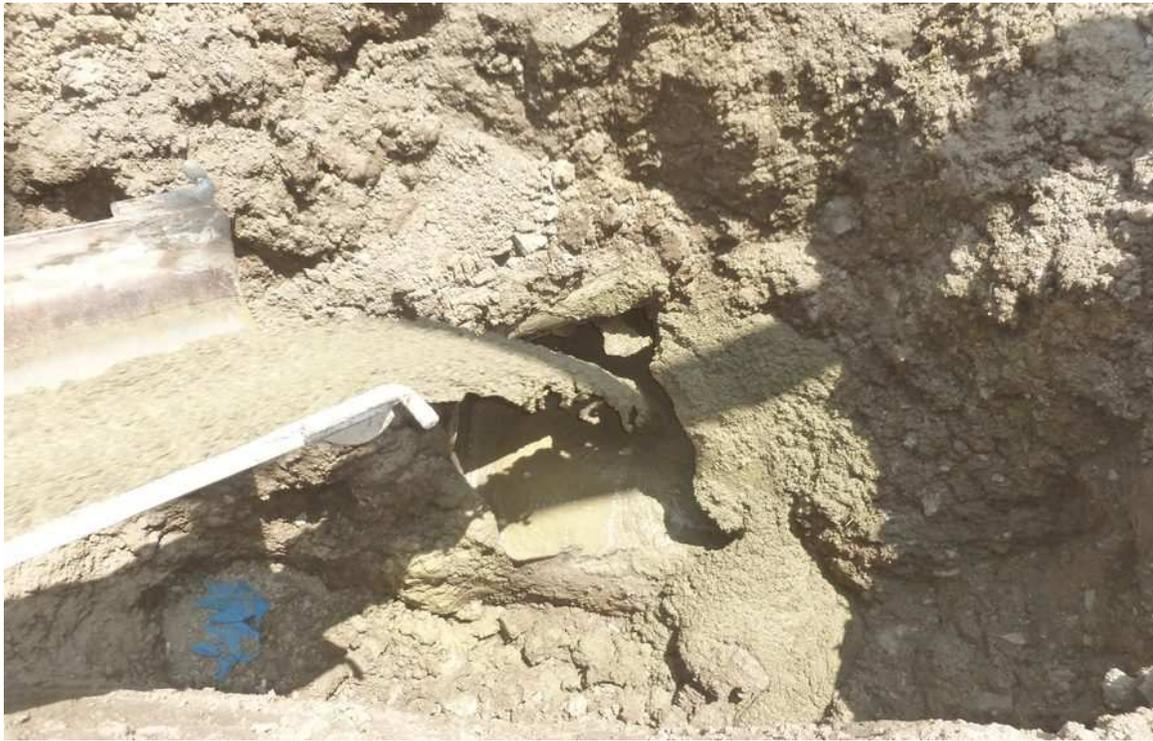
**Photo # 5. Filling the UST with 5.5 yards of sand/cement slurry.**
