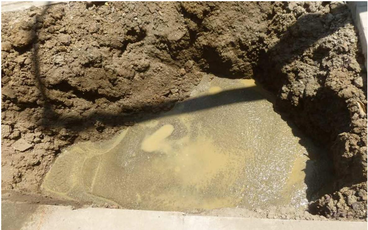
**Photo # 6. UST completely filled with sand/cement slurry.**
