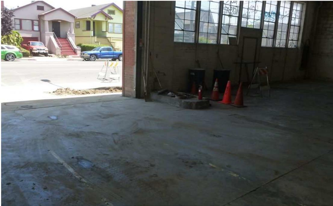
**Photo # 7. Dispenser pad with UST excavation on the other side of the building wall. This area is to be explored at the same time the groundwater confirmation samples are taken downgradient of the UST location.**
