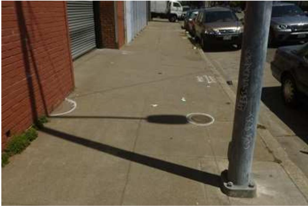
Subject: View of the UST fill port location. The UST extends towards the light pole, and approximately 50% of the tank is beneath the pole.
