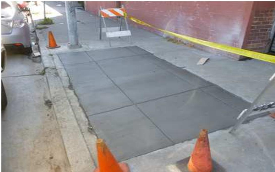
**Photo # 8. Finished sidewalk repair.**
