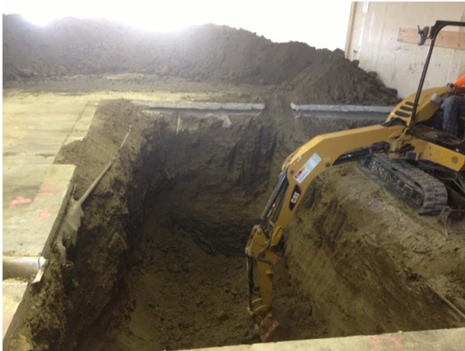
Photo #4: View of the general excavation area at 7104 tenant space prior to backfilling with concrete slurry. Excavator is located atop completed slot excavation area.
