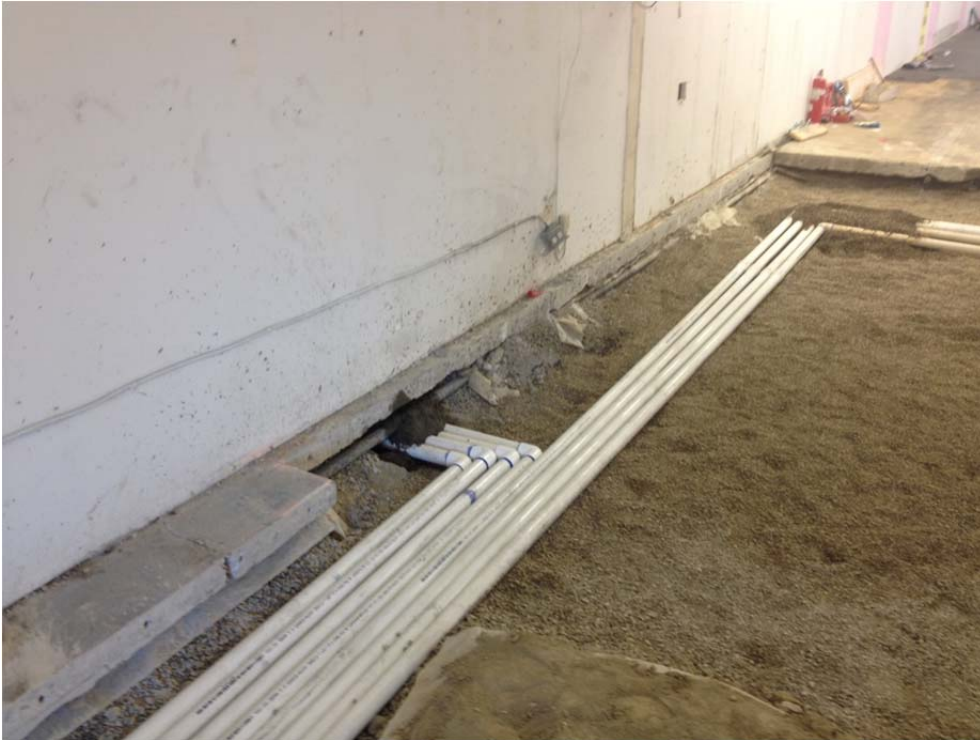
Photo #7: Sub-slab depressurization system through shear wall from the 7102 tenant space into the 7104 tenant space.
