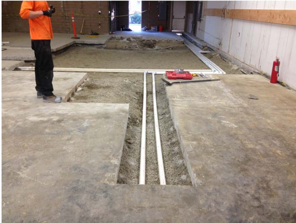
Photo #5: View of sub-slab depressurization system piping on top of pea gravel at 7102 tenant space. Pea gravel was then placed atop the PVC piping per IRAP.
