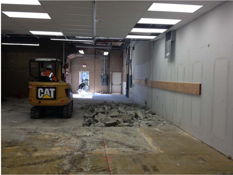
Photo #1: View of slot excavation area, concrete debris and shear wall bracing inside 7102 tenant space per IRAP.
