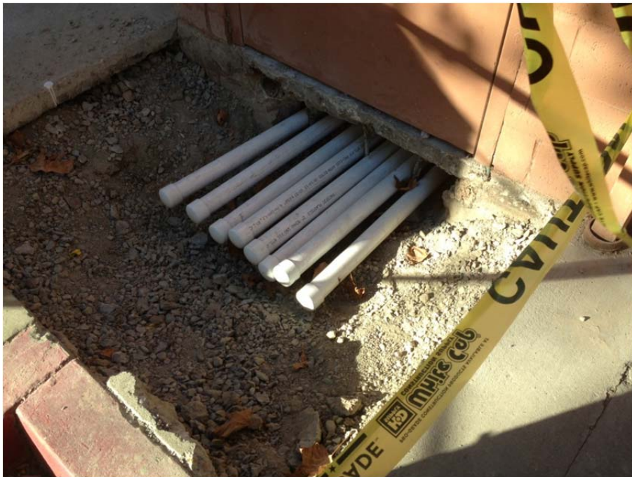
Photo #8: Sub-slab depressurization system and capped piping exiting building at rear of 7102 tenant space.
