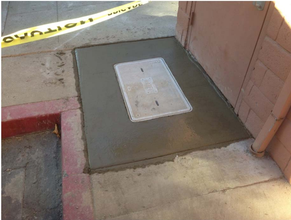
Photo #9: Completed sub-slab depressurization system vault box located at rear of 7102 tenant space.
