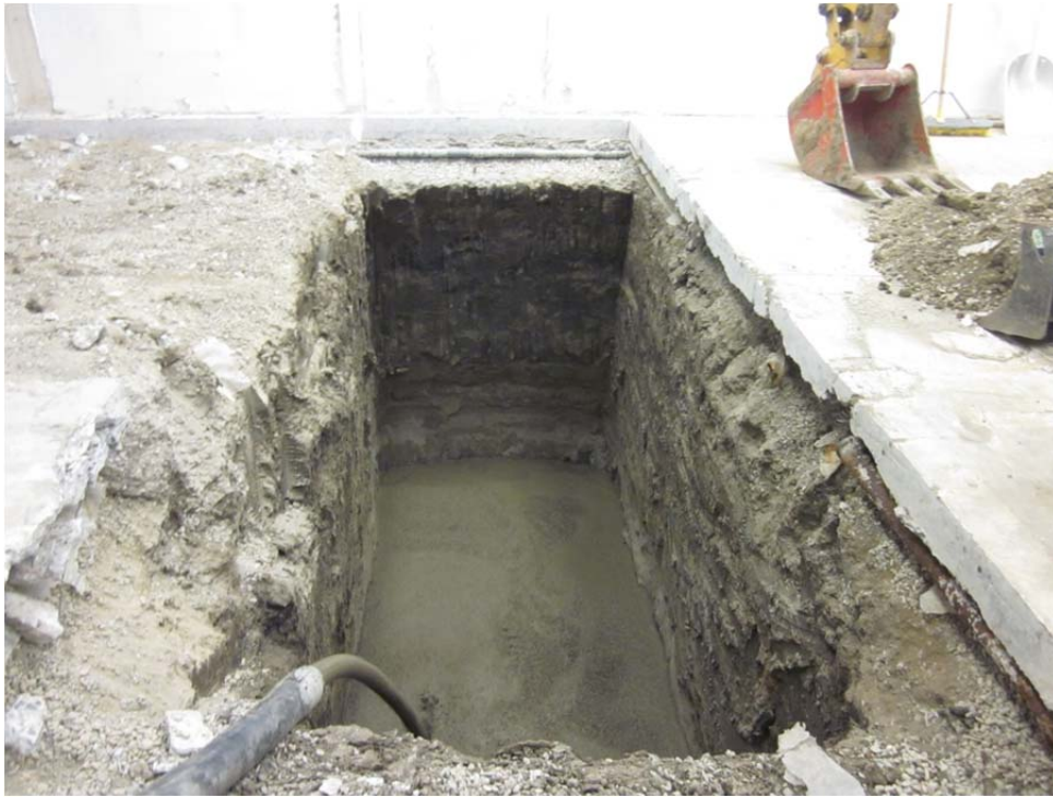
Photo #3: View of a slot excavation area in the 7102 tenant space being backfilled with concrete slurry.
