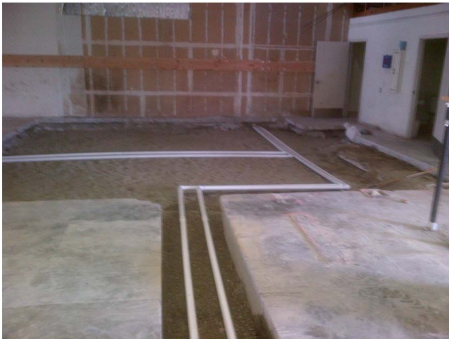
Photo #6: View of sub-slab depressurization piping on top of pea gravel at 7104 tenant space. Pea gravel was then placed atop the PVC piping per IRAP.
