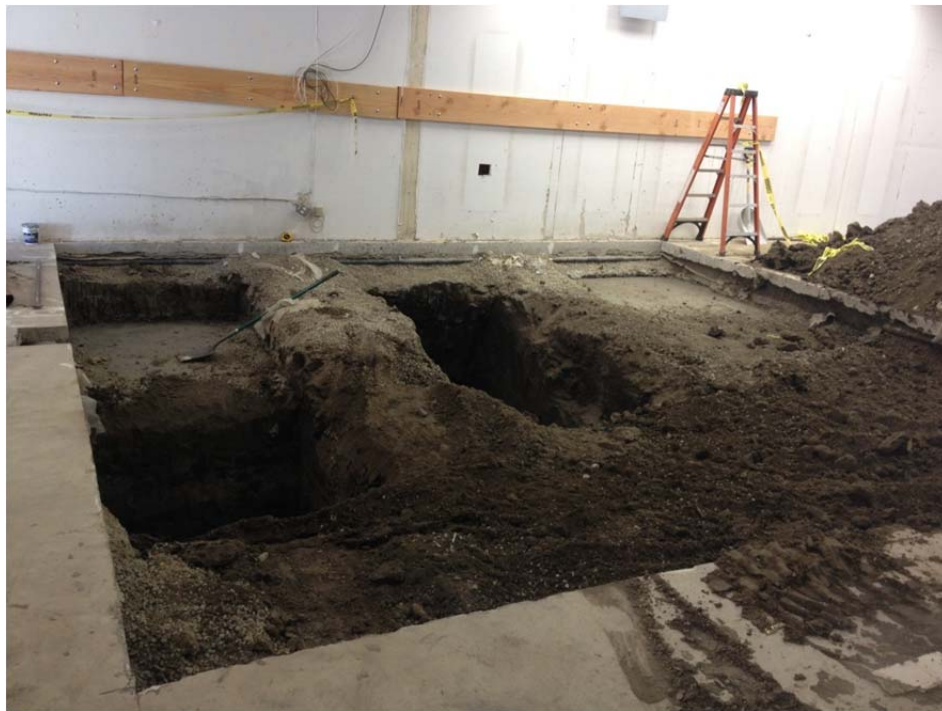
Photo #2: View of three slot excavation areas in 7102 tenant space with shear wall bracing per IRAP. The other two slot excavation areas between these areas were completed when the concrete slurry fully cured.
