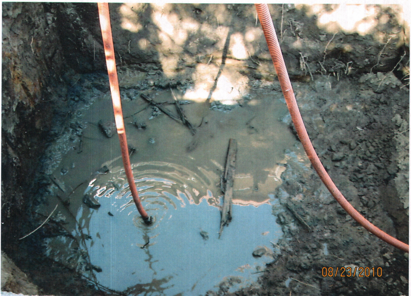
8/23/10 San Lorenzo USD UST Removal Water being sucked out of the pit.
