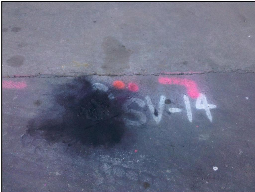
**PHOTO 8:** Typical surface patch after abandonment (concrete dyed black).
