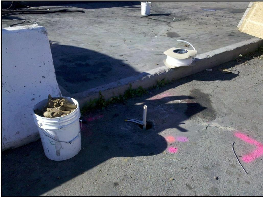
**PHOTO 1:** Overview of SB-1 after water sample collection and prior to grouting.
