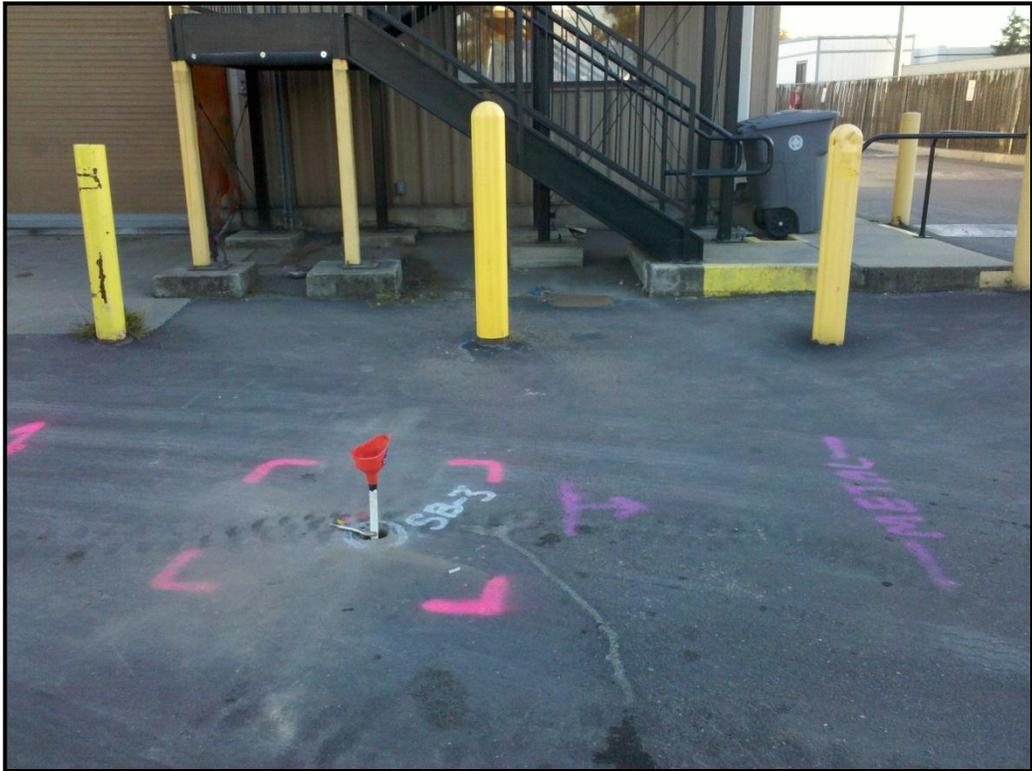
**PHOTO 5:** Grouting SB-3 after sampling.
