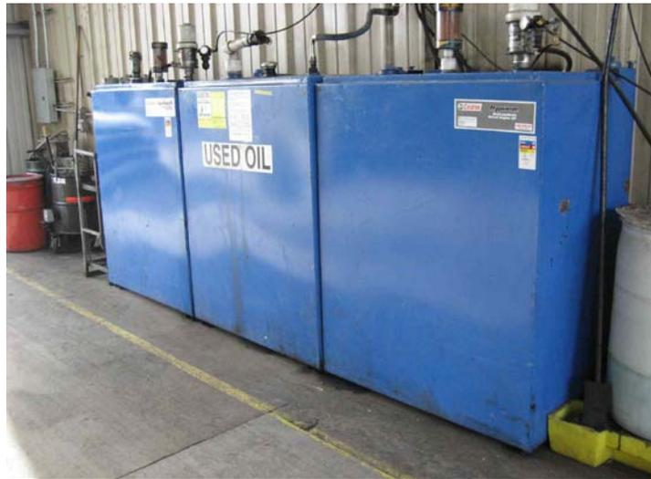
Photo 18: 350-Gallon Motor Oil, Waste Oil, and Transmission Fluid ASTs.
