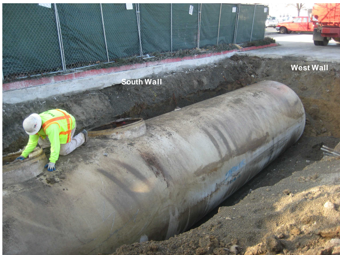
Tank Pit TP2 and Diesel Storage Tank
