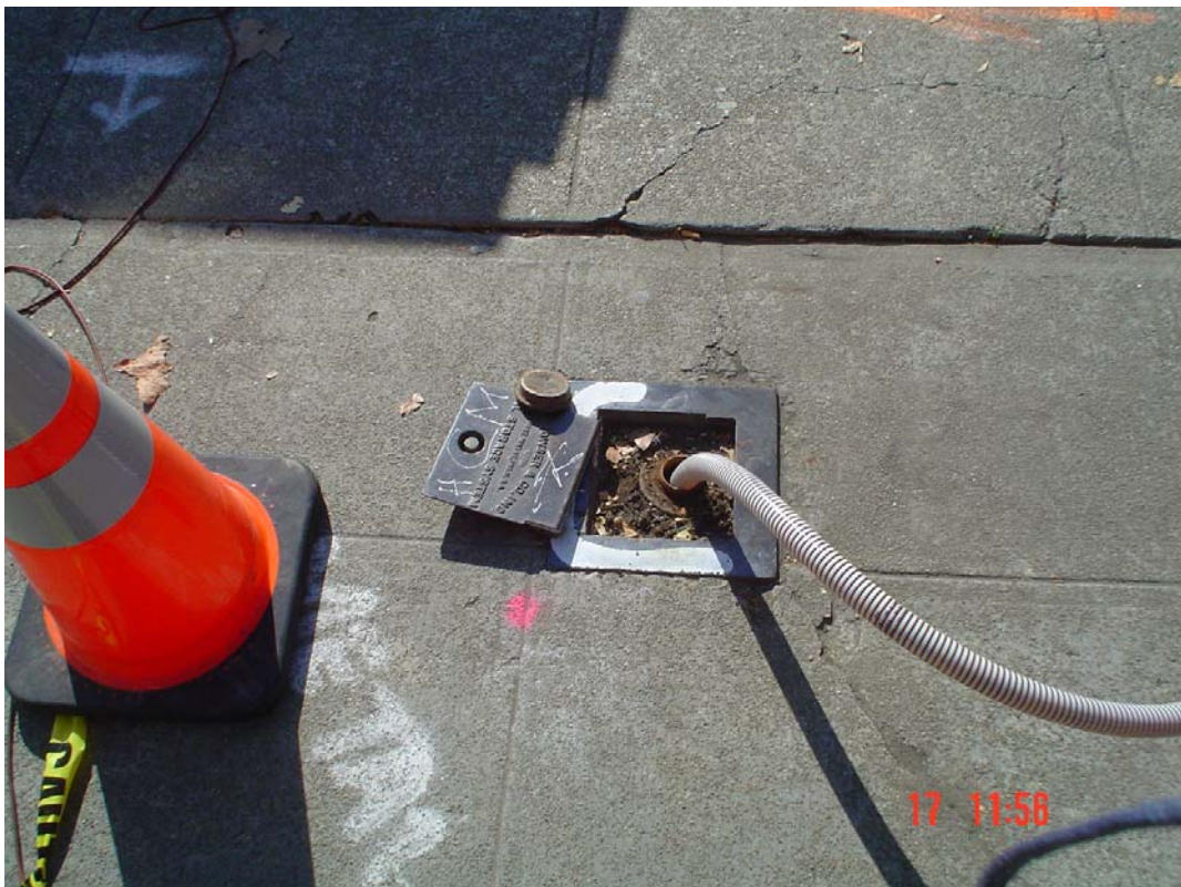
Plate 12: Decommissioning activities, tank purging and triple-rinsing
