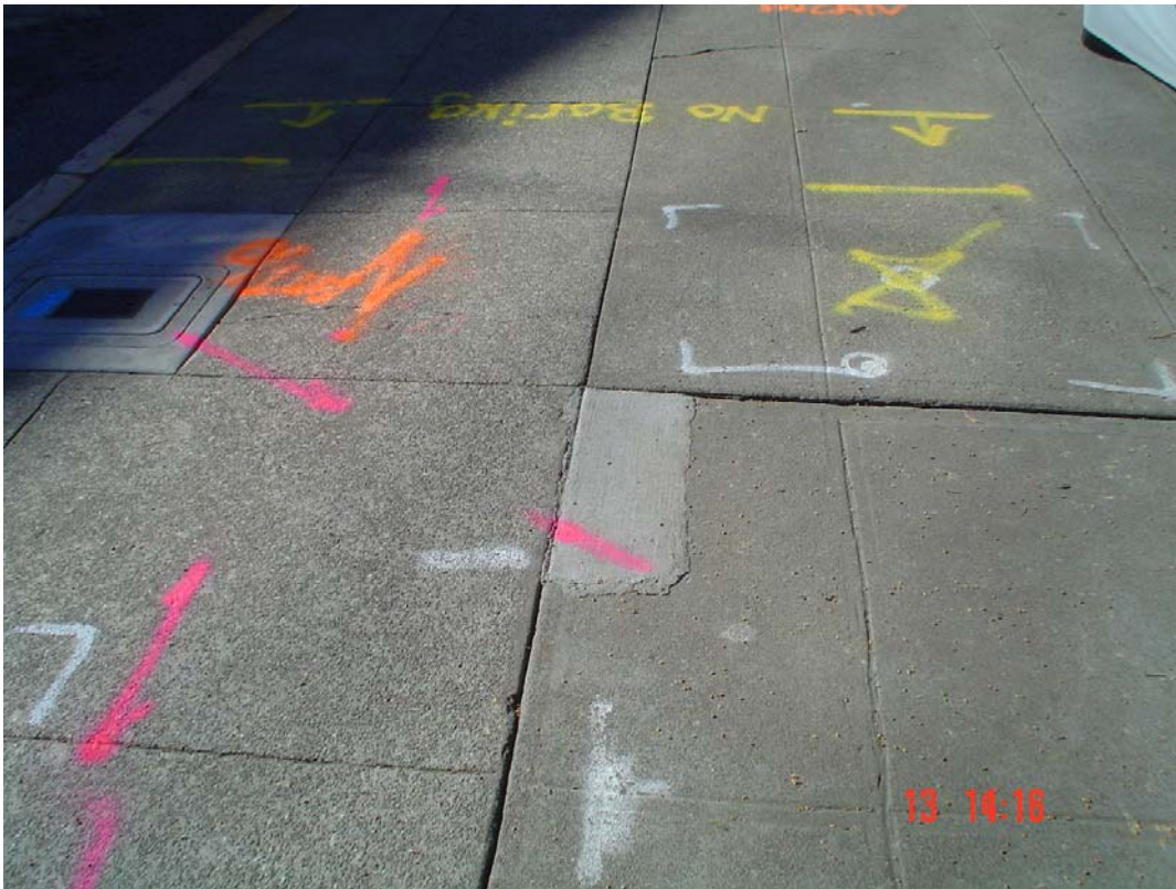
Plate 9: "No boring" signs and utility lines markings next to Tank 2
