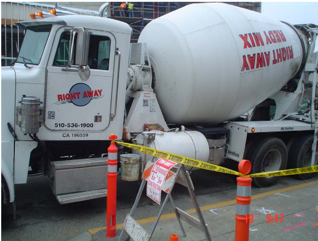
Plate 13: Decommissioning activities, cement truck with slurry mix
