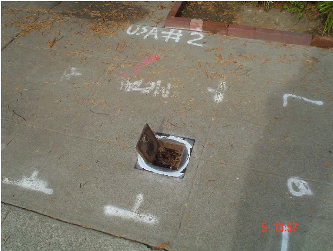
Plate 3: Small fill port (Tank 2)
