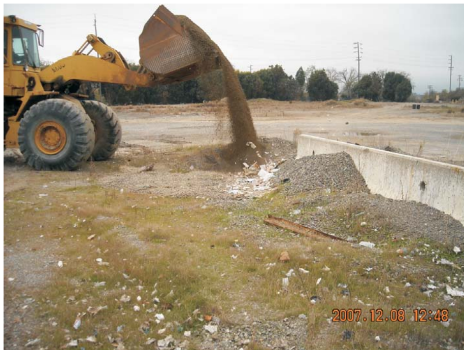
Eastern Conveyor Entrance Post Abandonment
