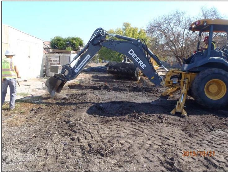
**PHOTO 33:** Additional excavation west of SW-5 on October 21, 2013, looking to the southeast. Water application for dust control.
