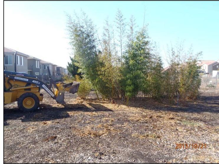
**PHOTO 34:** Removing bamboo in preparation for excavation in the southwest portion of 24137 Eden Ave.
