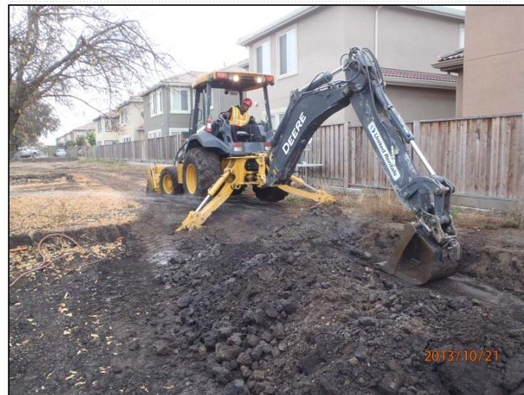
**PHOTO 32:** Additional excavation south of SW-17 on October 21, 2013, looking to the southeast. Water application for dust control.
