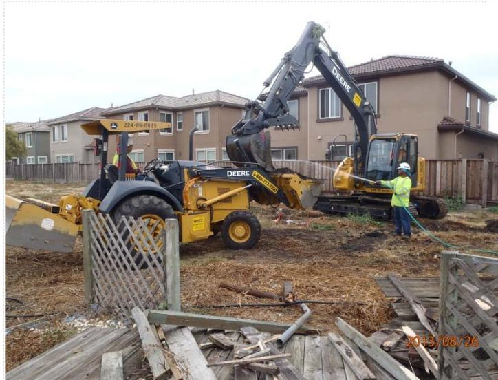
**PHOTO 8:** Transferring excavated soil from excavator to loader. Water application for dust control. Looking to the southwest.
