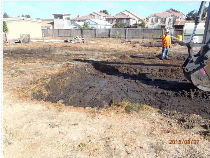
**PHOTO 14:** View of 36-GS12 area during excavation with water application for dust control.
