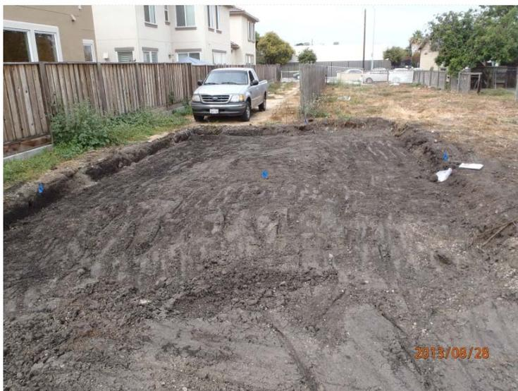
**PHOTO 17:** 36-GS8 after completion of excavation and confirmation sampling, looking to the west. Blue flags mark sampling locations.
