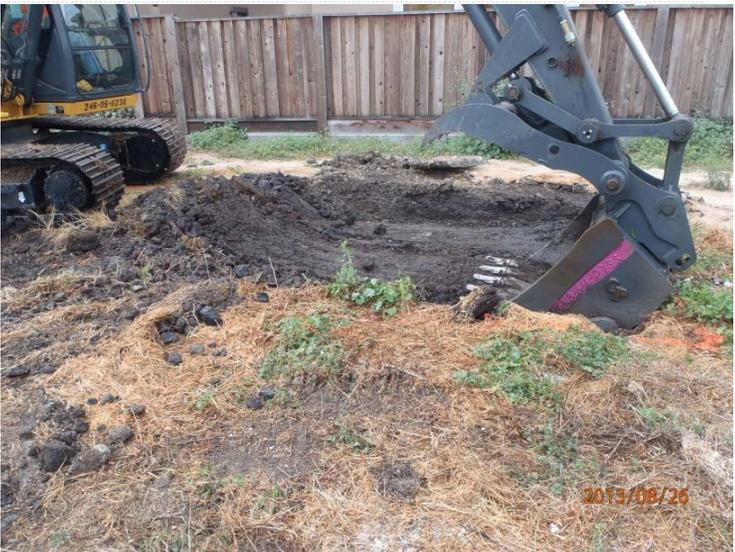
**PHOTO 7:** Excavation of 36-GS8 area. Soil was placed in stockpile for disposal at Class 1 facility. View to south.
