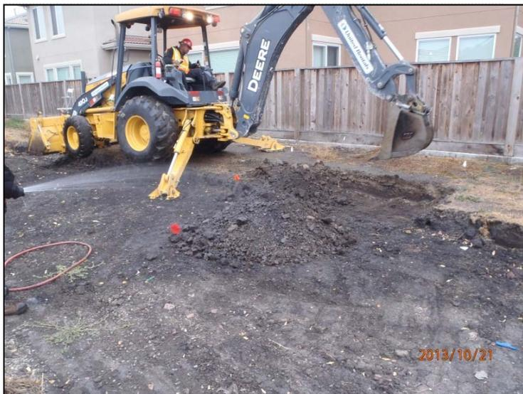
**PHOTO 31:** Additional excavation south of SW-9 on October 21, 2013, looking to the south. Water application for dust control.
