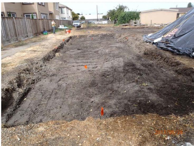
**PHOTO 19:** 36-GS12 and 36-GS13 areas after completion of excavation and confirmation sampling, looking west. Flags mark sampling locations.
