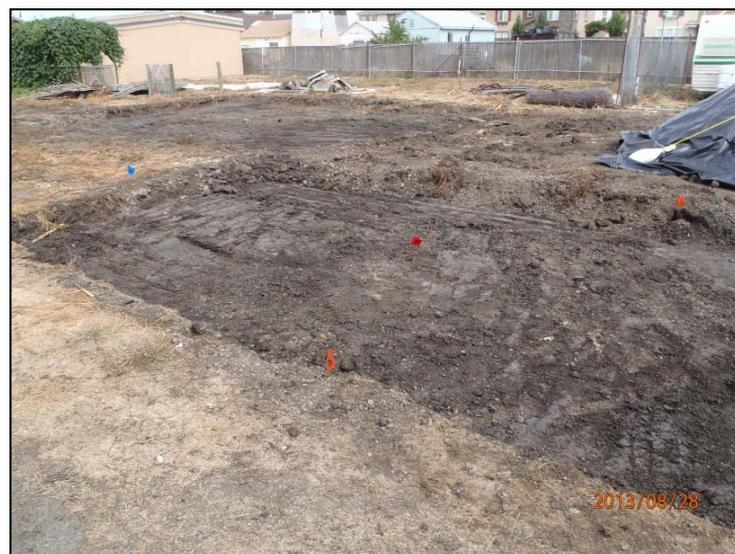
**PHOTO 18:** 36-GS12 and 36-GS13 areas after completion of excavation and confirmation sampling, looking to northwest. Flags mark sampling locations.
