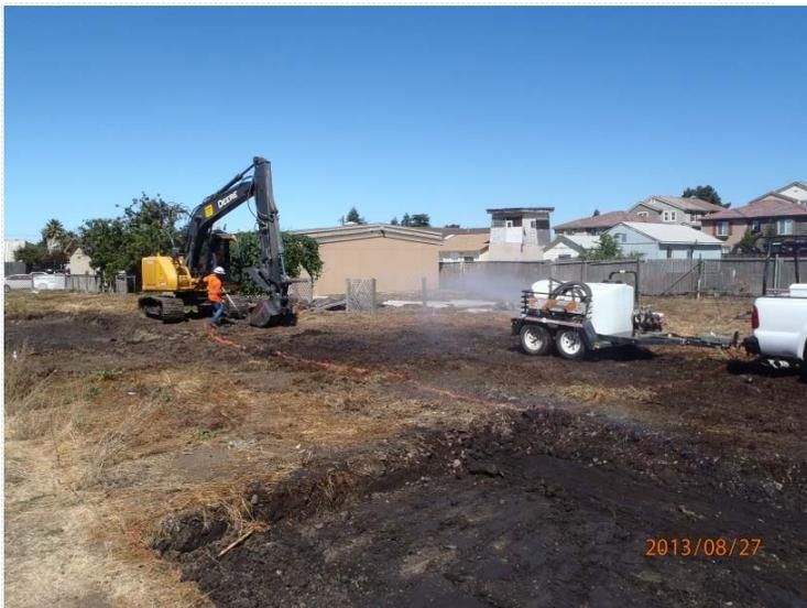
PHOTO 11: Pre-watering for dust control prior to excavation.
