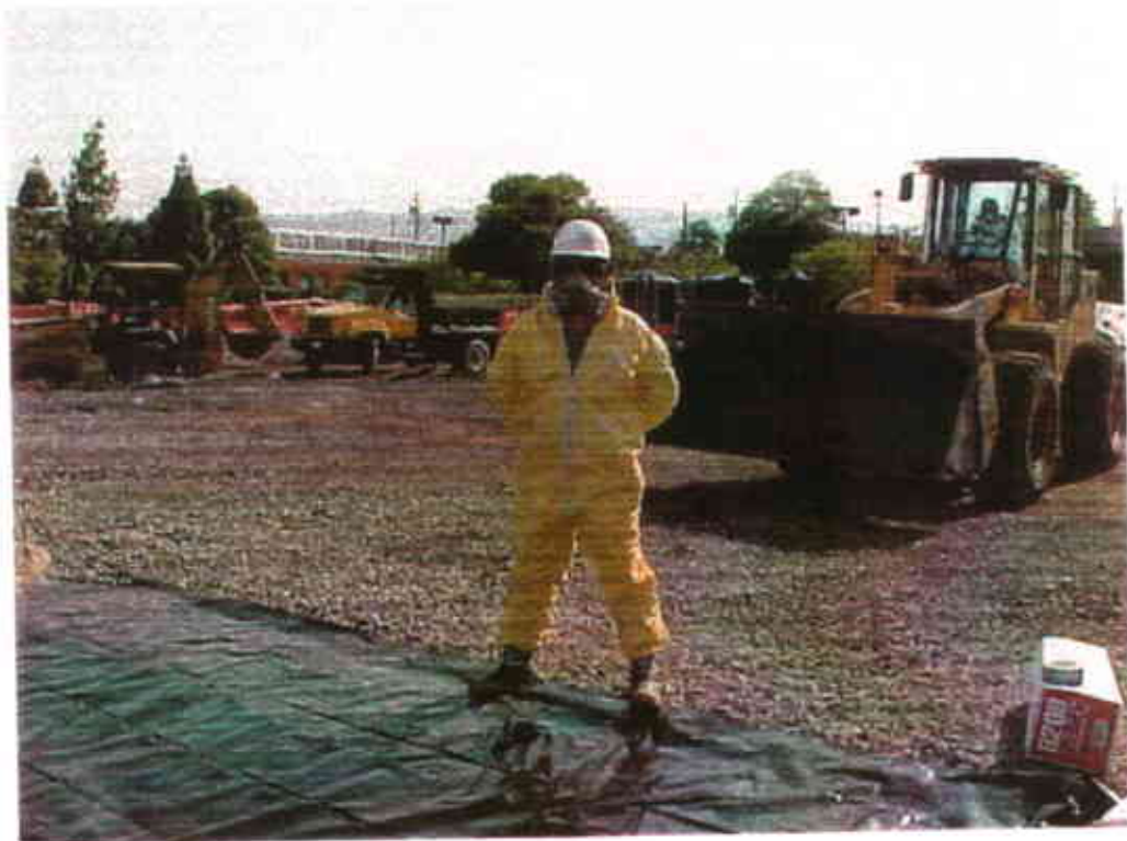
Figure A4. Personal Protection Equipment during excavation activities
