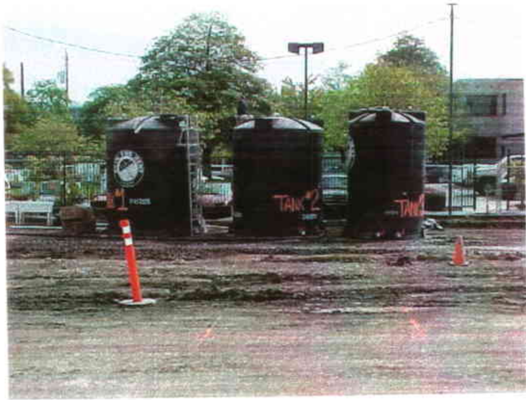
Figure A3. De-watering and storing purged groundwater in tanks
