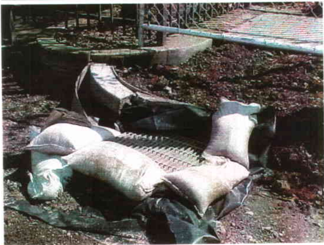
Figure A7. Protection of storm drains
