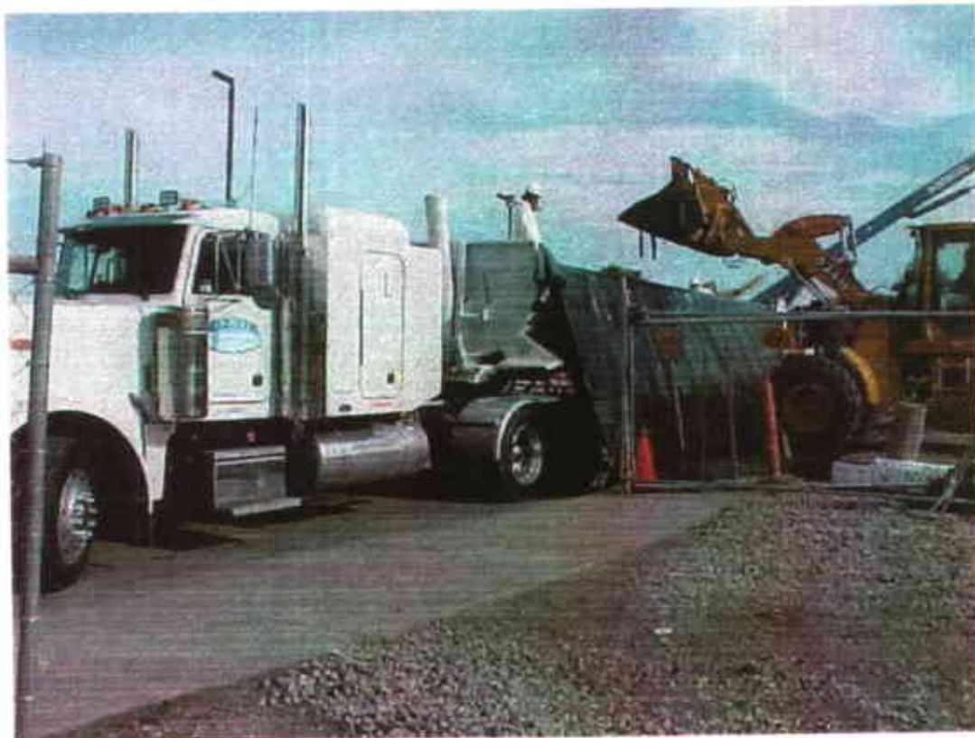
Figure A6. Loading contaminated soil to trucks
