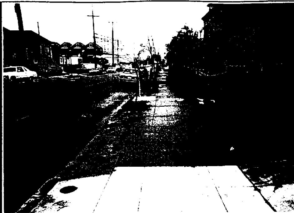
VIEW SOUTHWEST DOWN THE NORTH SIDE OF 64TH STREET WITH THE SUBJECT PROPERTY IN THE FOREGROUND
