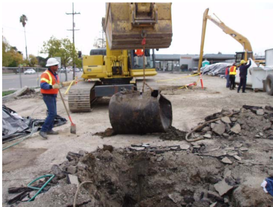
Photograph #2: Tank as it is being removed from the ground. The hole located at the top right corner was caused during excavation activities, prior to knowledge of the tank.
