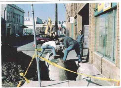
Subject: Inerting the tank by emplacing dry ice prior to disposal transportation.
