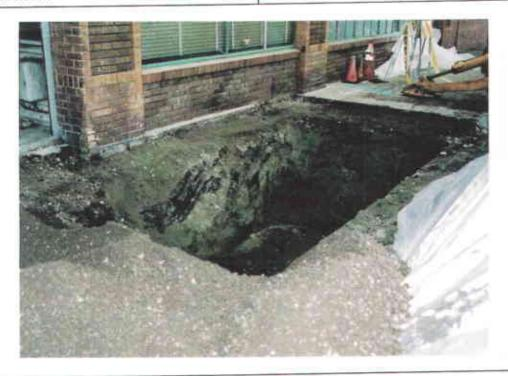
Subject: Open excavation after removal of tank and collection of confirmation samples.
