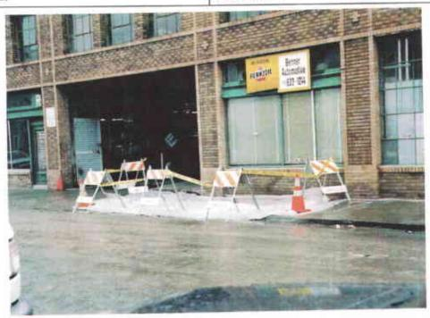
Subject: Location of former tank. SES scope of work completed. Excavation is backfilled and awaits concrete pouring.
