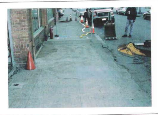
Subject: Location of UST under sidewalk in front of Benner Automotive. Note cold-poured concrete from tank installation.
