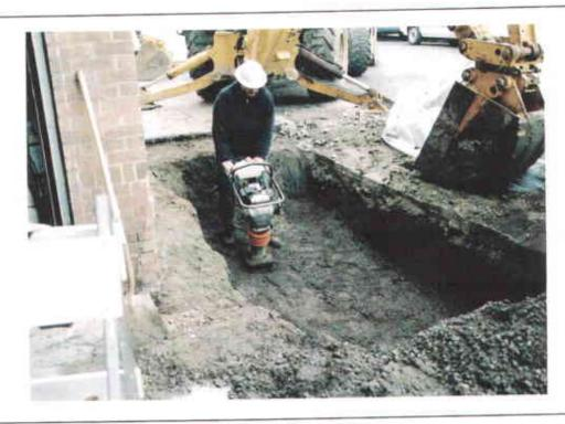
Subject: Compacting backfill in excavation to meet City of Oakland requirements.
