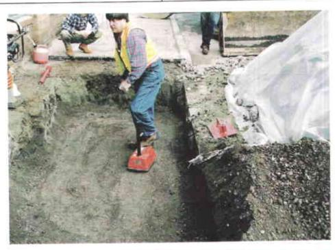
Subject: Mark Hopkins of Construction Materials Testing, Inc. testing backfilled excavation to ensure 95% compaction.
