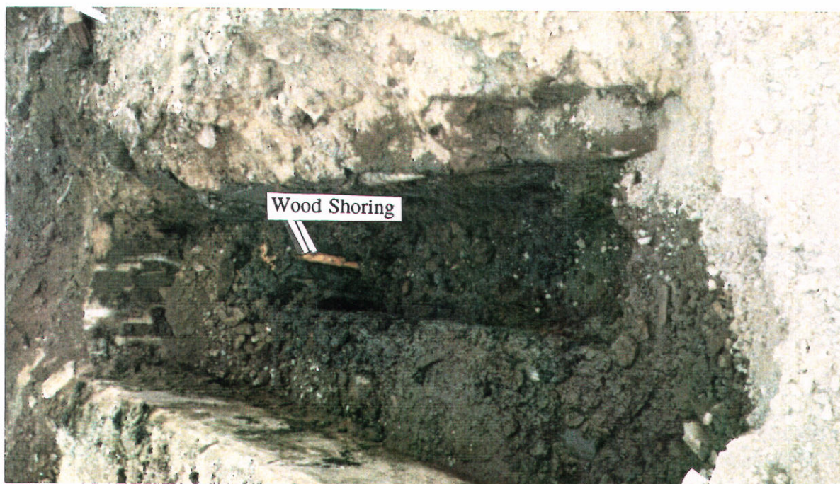
B. (Looking west) wood shoring visible during early excavation activities, 31 August 1995.
