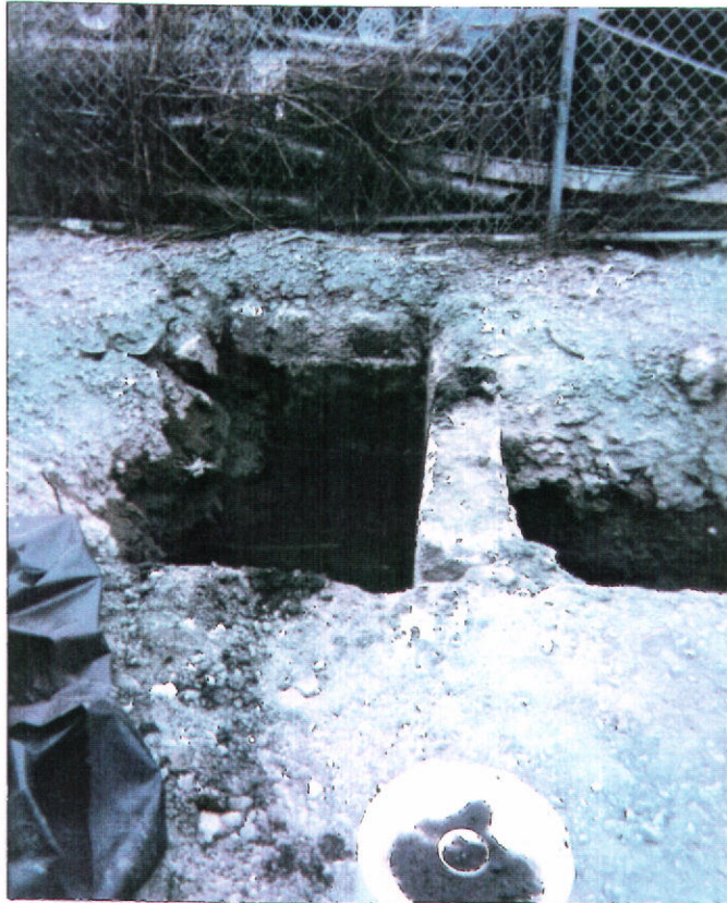
A. (Looking northeast) view of concrete-lined sump and portion of discharge tunnel trench to the right, 11 September 1995.
