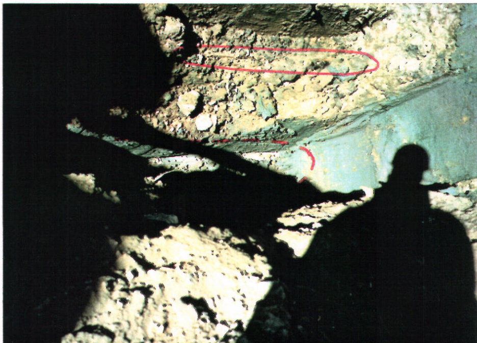
A. (Looking southwest) view of concrete top of discharge tunnel (dashed circle), outline of wood shoring (solid circle) along south trench wall, 28 August 1995.
