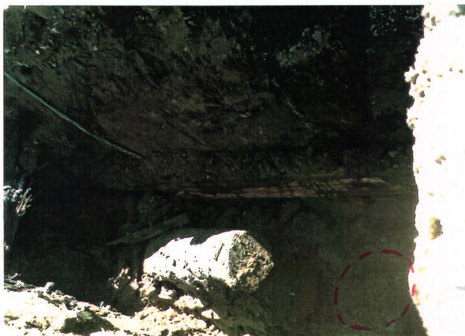
B. (Looking south) view of wood shoring along south trench wall, and concrete top of discharge tunnel at bottom of trench (circled), 28 August 1995.
