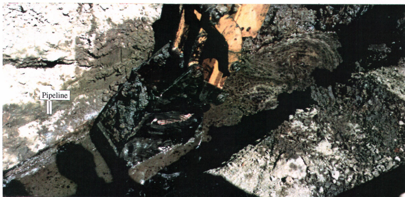
A. View of groundwater in discharge tunnel during high tide; product and an oily sheen visible on groundwater surface, 31 August 1995.
