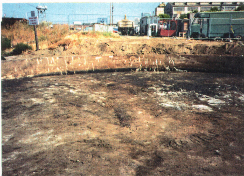
E. View of northern portion of excavated concrete containment.
