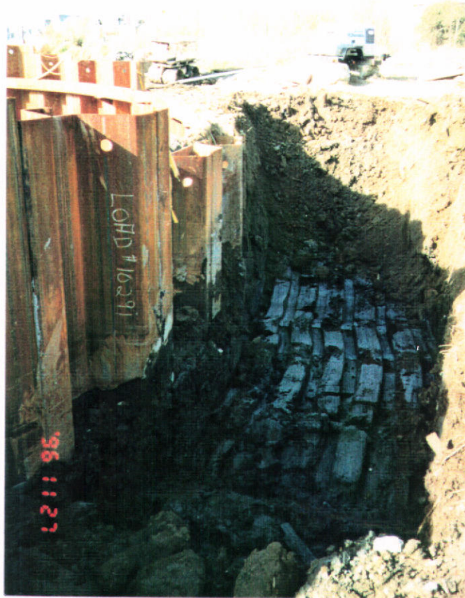
Trench on the northern side of the former containment structure.
