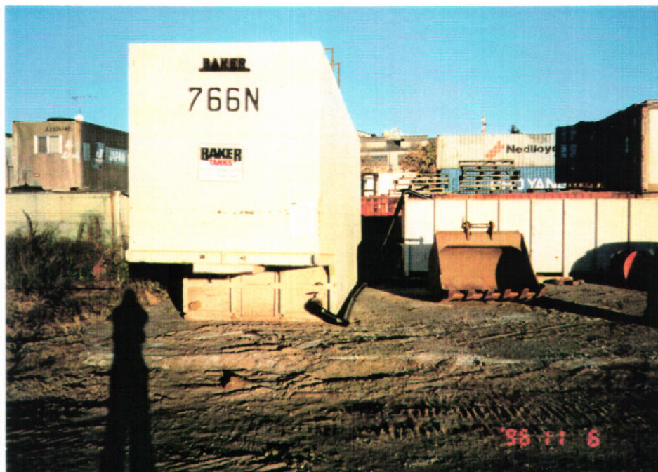
Dewatering storage tank (left) connected to treatment tank (right) with black PVC piping.
