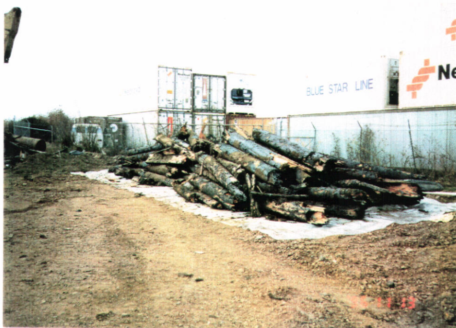
Wood pilings removed from excavation area.
