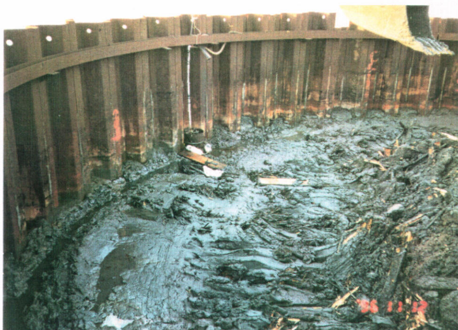
Limits of excavation showing Bay Mud and dewatering sump (center).
