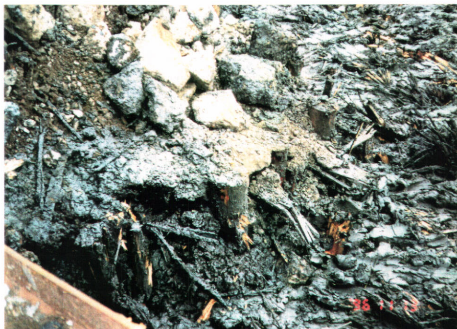
Typical wood pilings at face of excavation.
