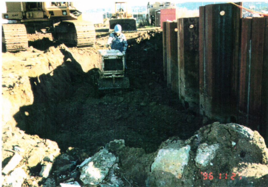
Backfilling and compaction of the trench on the northern side of the former containment structure.
