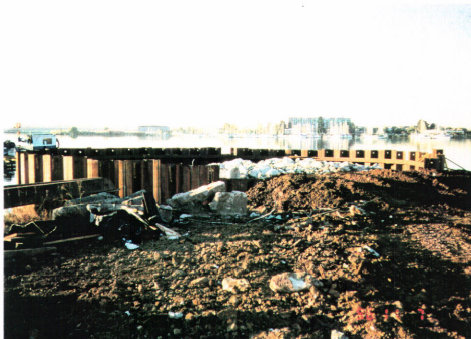
Sheetpiling surrounding excavation area with concrete rubble area used as equipment pad in center.
