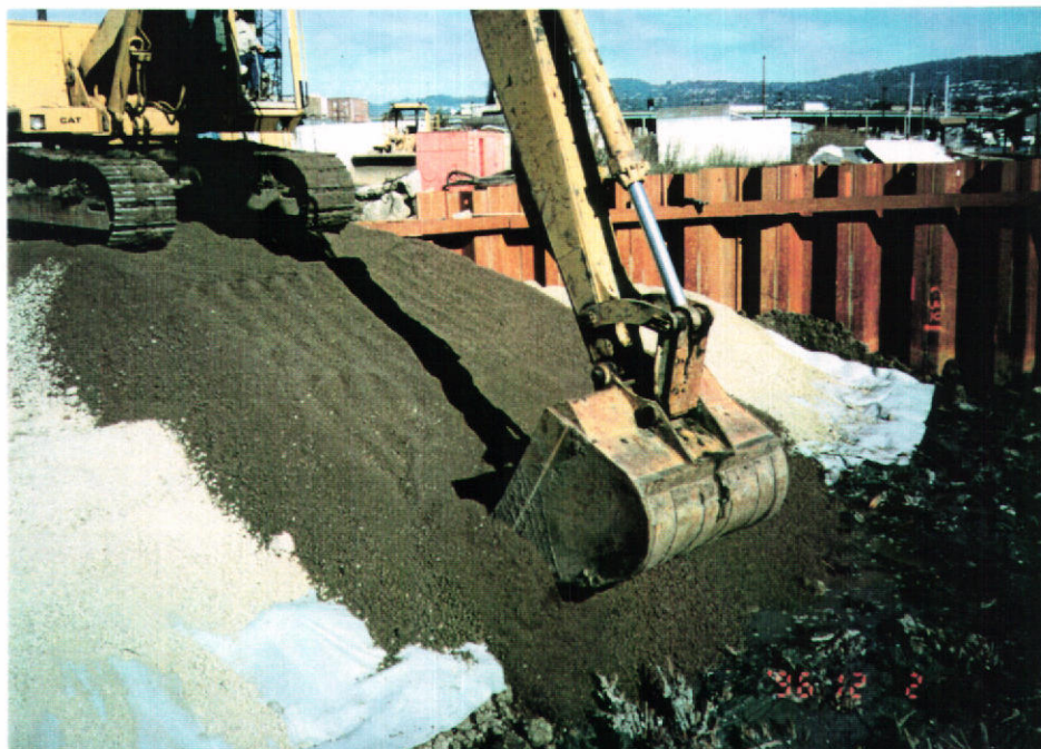
Backfill showing filter fabric, fine-grained fill (white), and coarse-grain fill (brown) being placed in excavation area.
