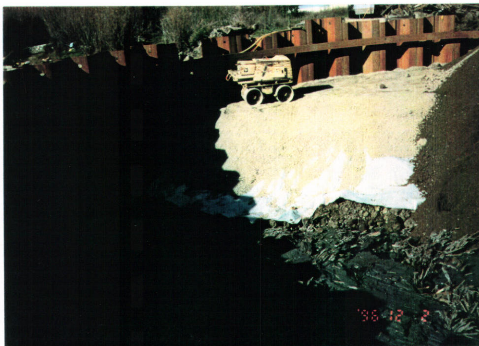
Compaction of fill material over filter fabric.
