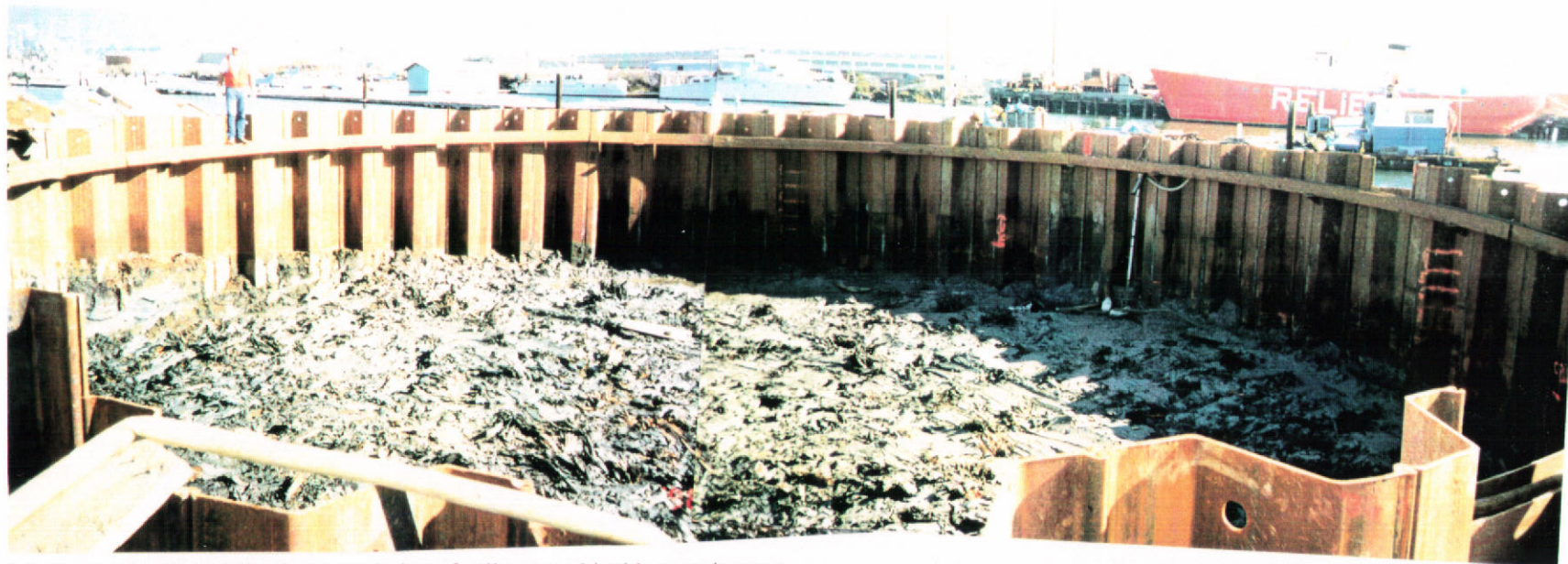
Limits of excavation following completion of soil removal inside containment.
