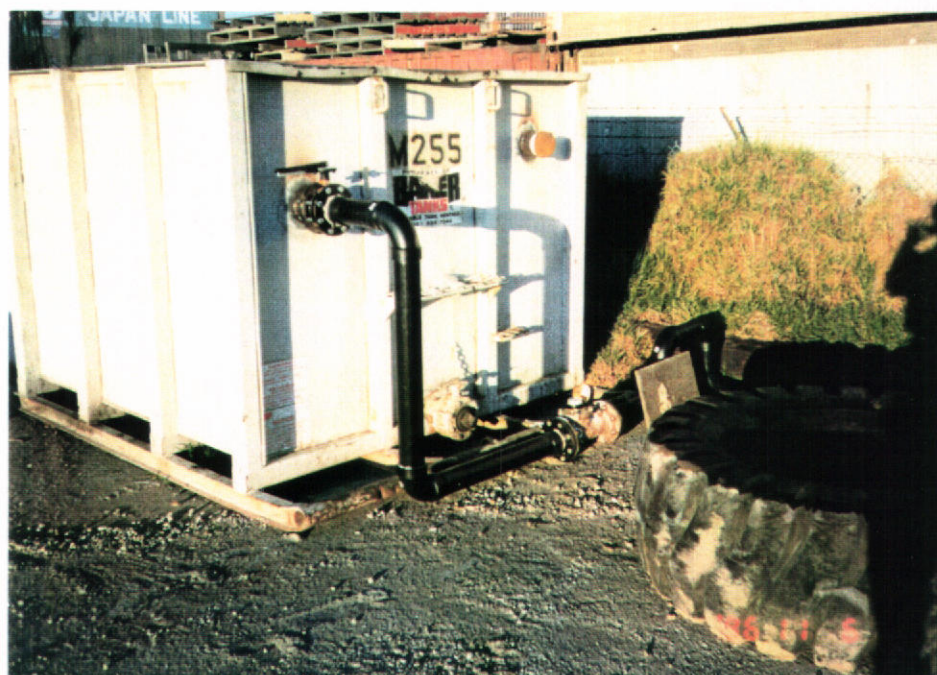
Discharge end of treatment tank showing flow meter and discharge pipe.
