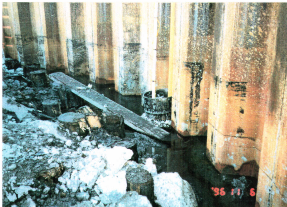
Dewatering sump and wood piling prior to excavation.
