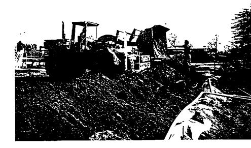
Loader places soil in stages. Vented pipe is laid horizontally near the base of the cell. A vertical "riser" connects two sections of horizontal pipe.
