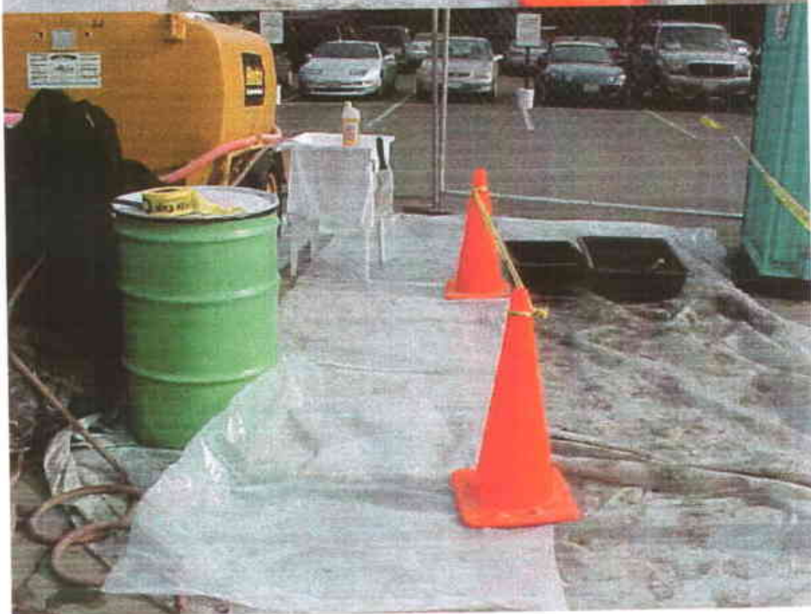
Worker Decontamination Area
