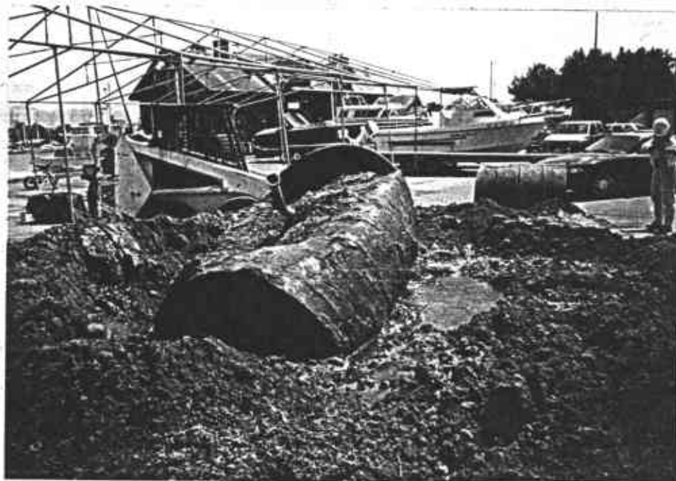
5) View of tank T2, partially crushed by excavator; fluid from tank ponded in stockpile.
