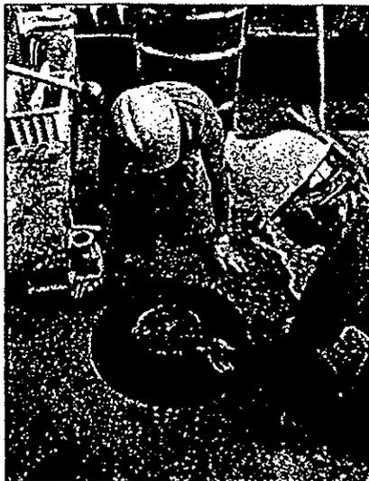
Finally, concrete around the well cover is trowelled smooth.
