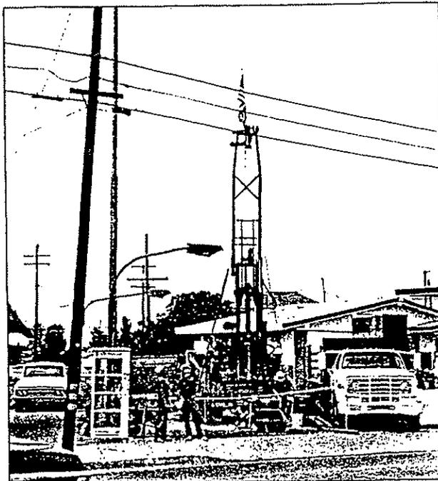
With city drilling you are close to power lines on adjacent streets. Service stations often are located on corner lots with overhead lines on two or three sides of the drilling site.
