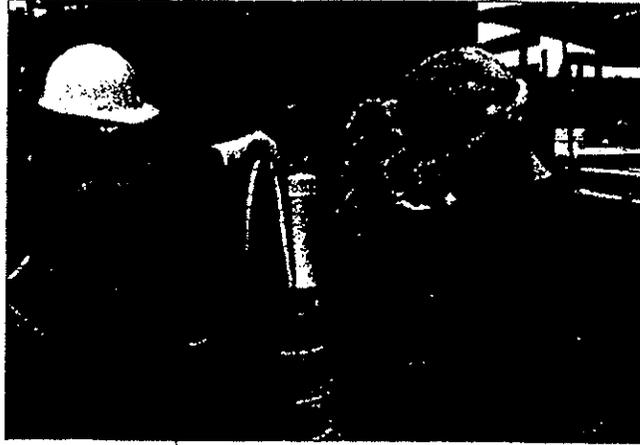
First, the space between the P.V.C. casing and the drilled hole is filled with sand, bentonite and cement grout to keep water from seeping into it.
