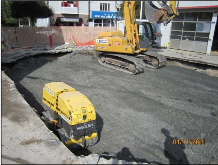
PHOTO 49: Compacting clean import fill above 4-feet.
