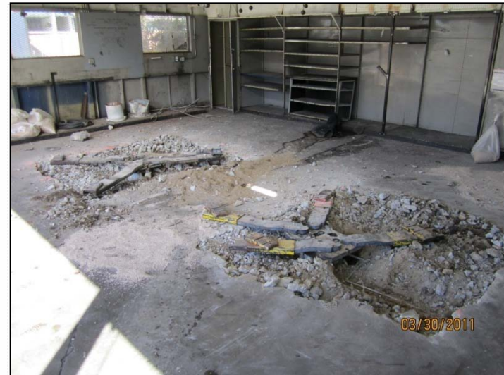
PHOTO 8: Concrete demolition completed around both hoists.
