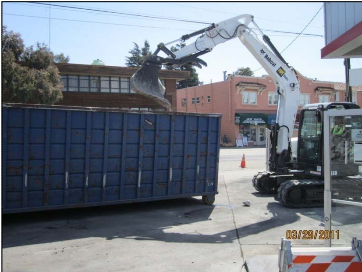
PHOTO 7: Loading processed concrete into debris bin.
