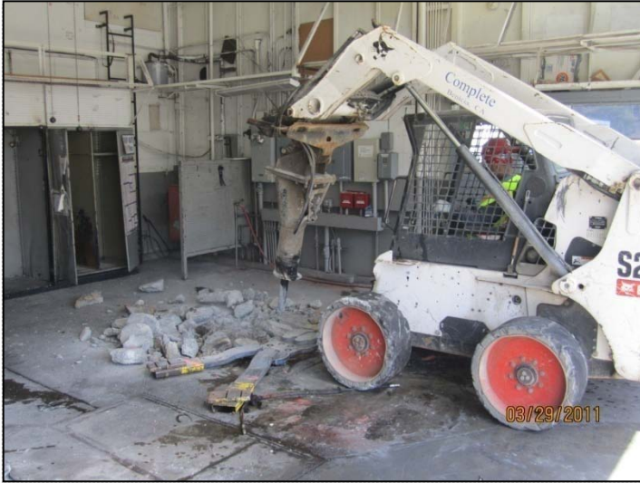
PHOTO 5: Breaking concrete around east hoist.
