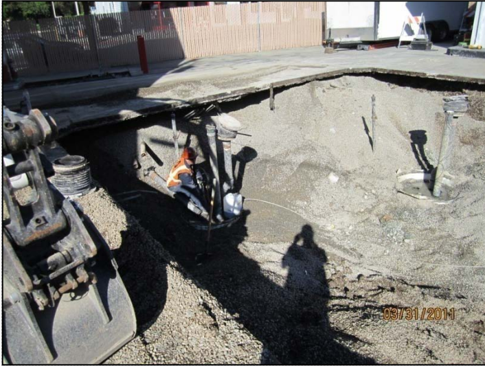
PHOTO 17: Steam cleaning 20K UST from fill end of tank.
