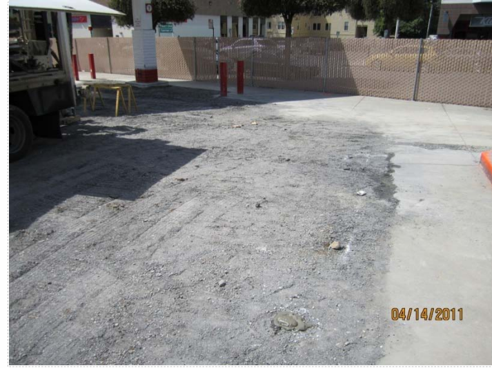
PHOTO 58: Boring UST1-C-18' after backfilling with neat cement.
