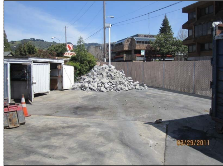
PHOTO 6: Processed concrete debris staged in the northeast tip of Site.
