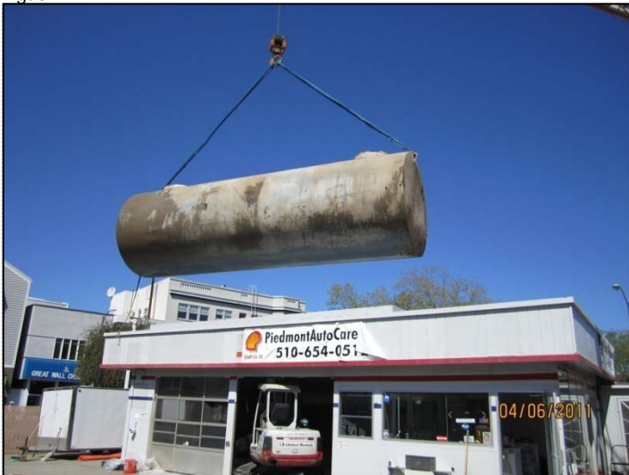
PHOTO 39: Clearing the station building with 20K UST.
