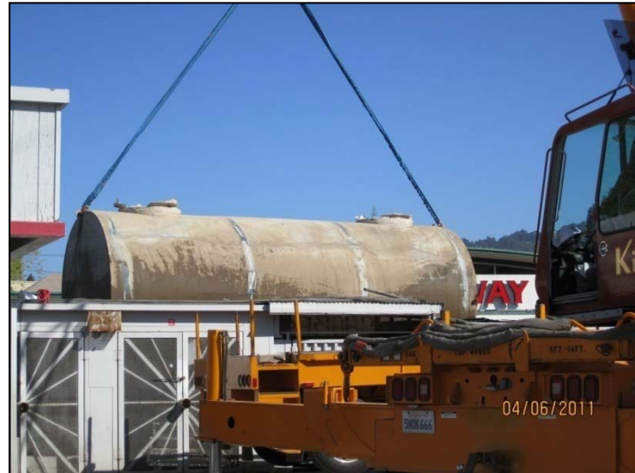
PHOTO 36: Setting down 15K UST on transport trailer.
