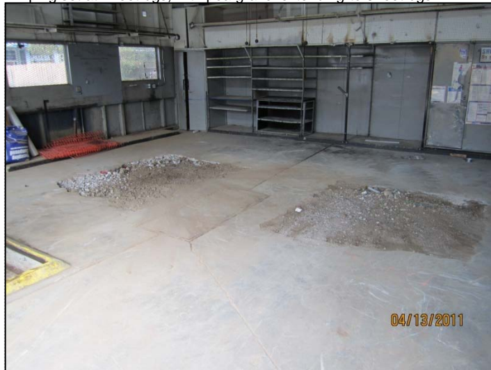
PHOTO 55: Hoist areas after removal and backfilling.
