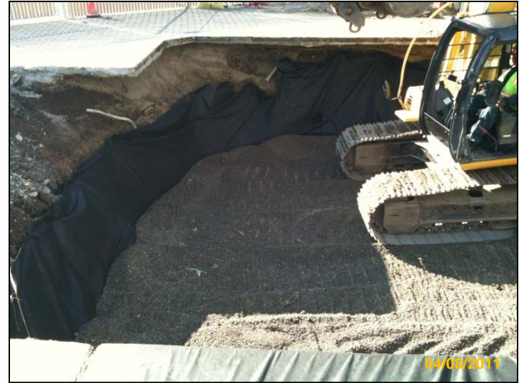
PHOTO 46: Compacting first layer of pea gravel on top of fabric.
