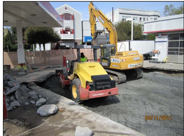
PHOTO 52: Compacting upper lifts with wheeled compactor.
