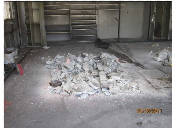
PHOTO 4: Concrete demolished around west hoist inside station building.
