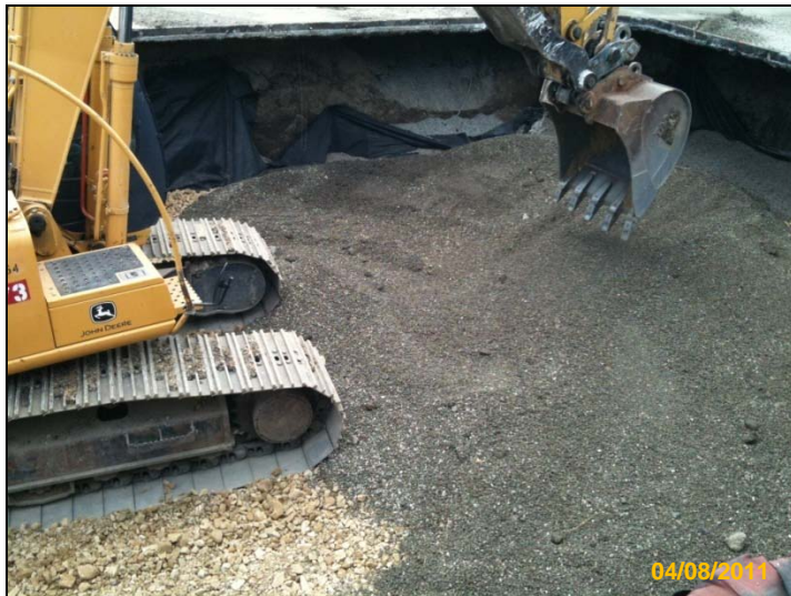
PHOTO 47: Adding base rock and second layer of pea gravel.
