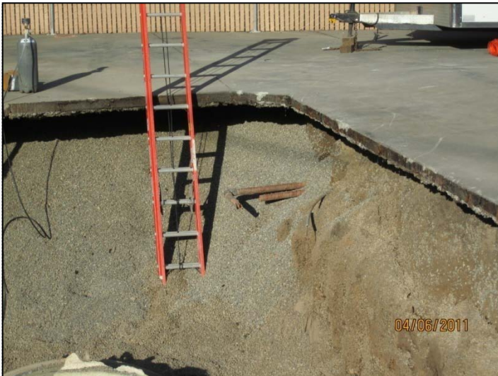
PHOTO 31: Looking at vent pipes in northwest corner of tank pit.
