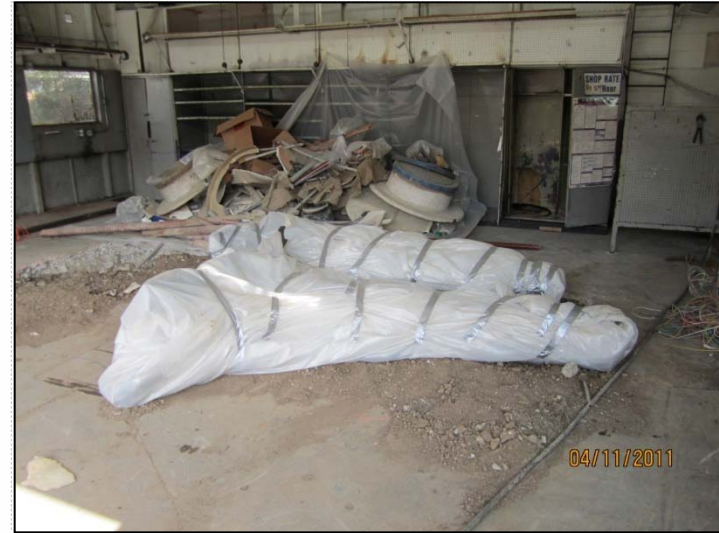
PHOTO 50: Hoists wrapped in plastic for off-site transport.
