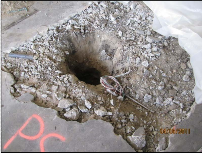
PHOTO 29: East hoist removed.
