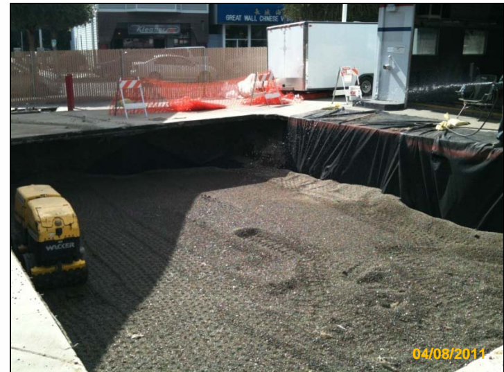
PHOTO 48: Compacting pea gravel with remote control vibrating compactor.
