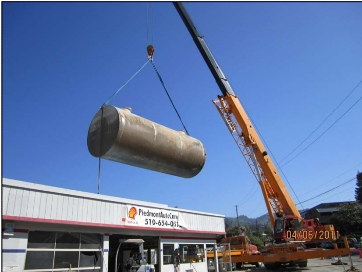
PHOTO 35: Lifting 15K UST over station building to awaiting flat-bed transport trailer.
