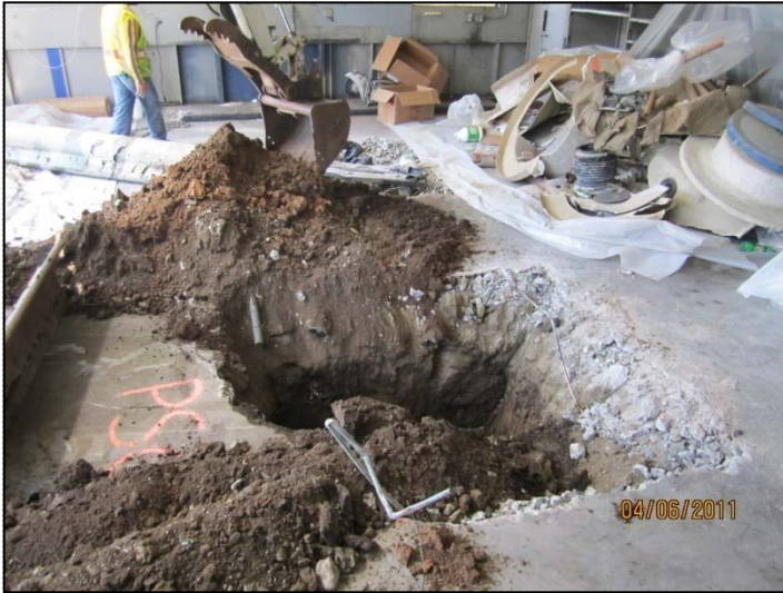
PHOTO 41: Excavating to base of east hoist (8 feet) for confirmation soil sample.
