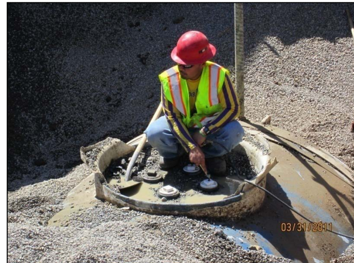
PHOTO 24: Adding 20 lbs of CO2 gas to 15K UST following triple rinse for preliminary tank inerting. A total of 60 lbs of CO2 gas was added to each tank, followed by dry ice, just before removal.
