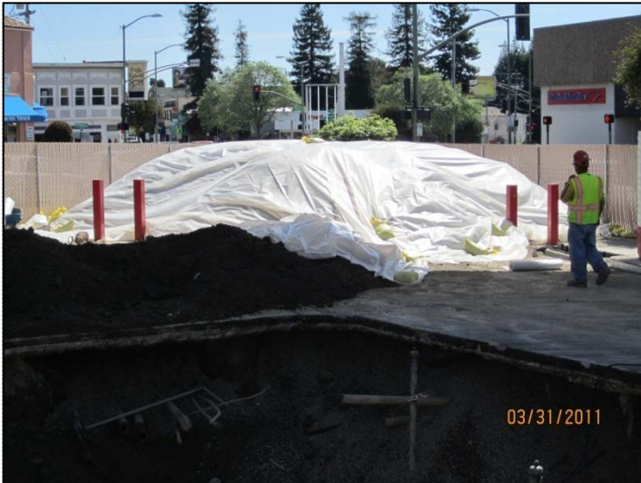
PHOTO 27: Approximately 200 cubic yards of pea gravel overburden covered with plastic.
