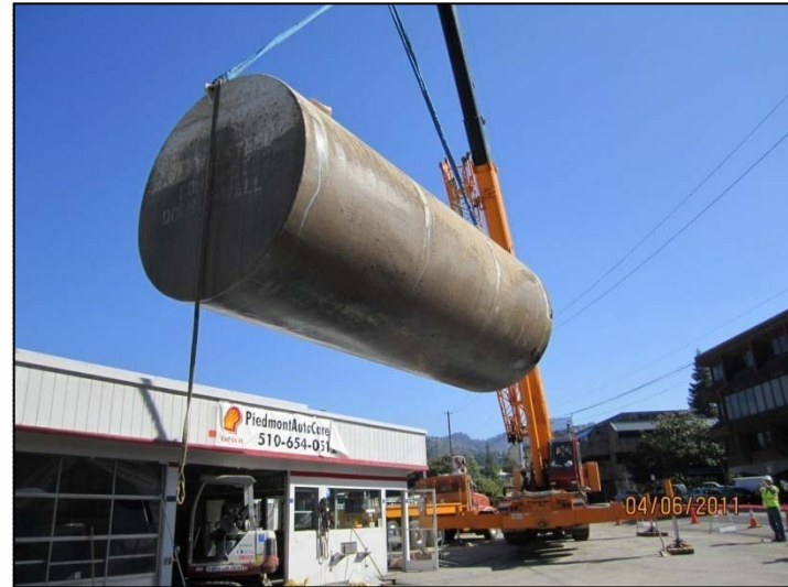
PHOTO 34: Raising 15K UST to clear station building.
