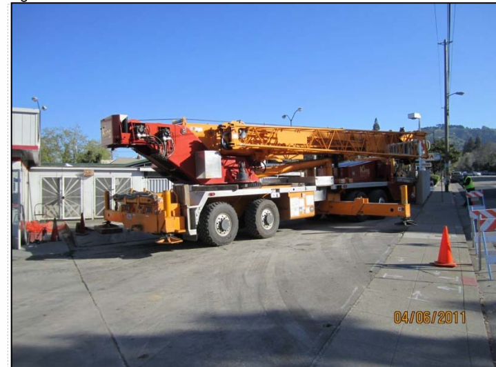
PHOTO 32: Setting up crane remove USTs,
