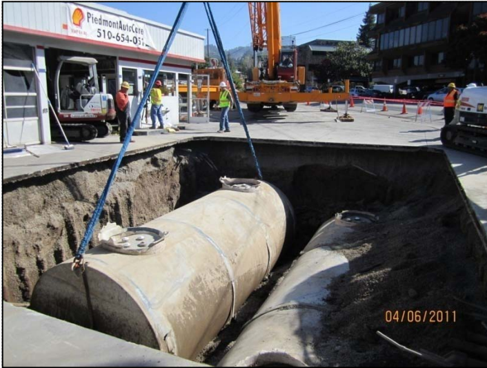
PHOTO 33: Picking 15K UST from pit .
