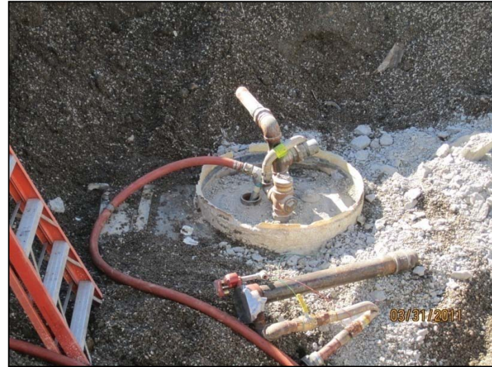
PHOTO 18: Steam clean rinsate vacuum recovery from pump end of UST.
