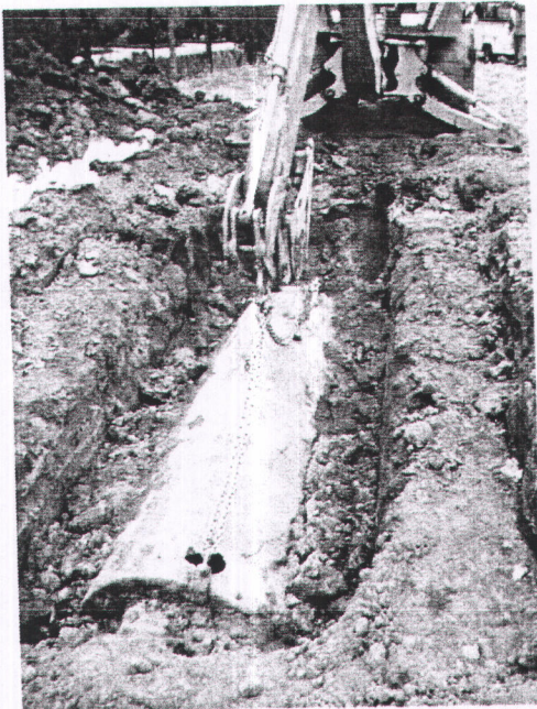
UST READY TO BE REMOVED FROM EXCAVATION
