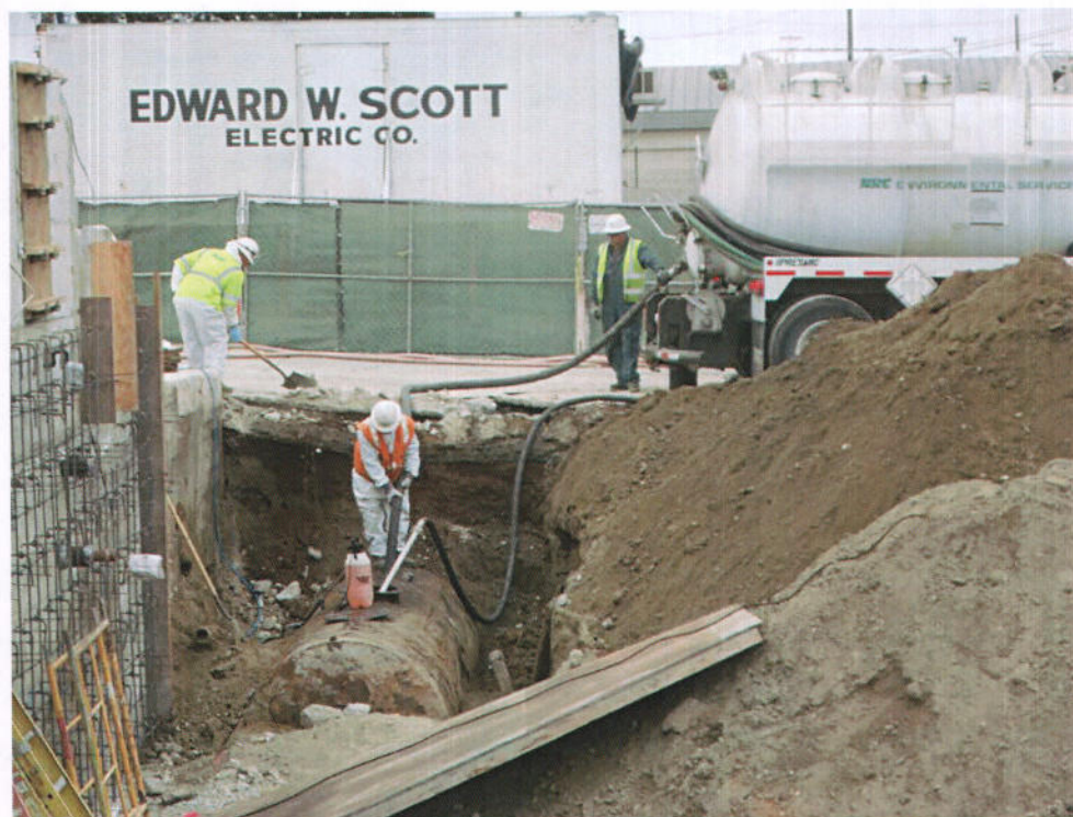
Photo 2 – View looking south as UST #1 is being cleaned.
