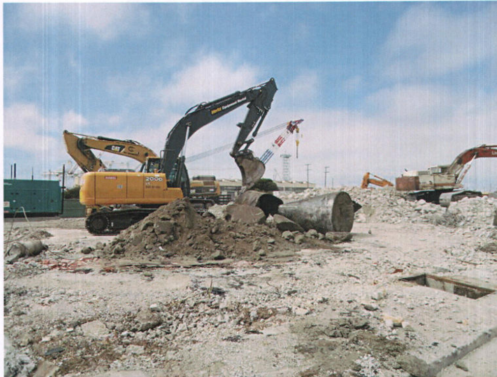
Photo 11 – View of UST #2 being smashed prior to removal from site as scrap metal.
