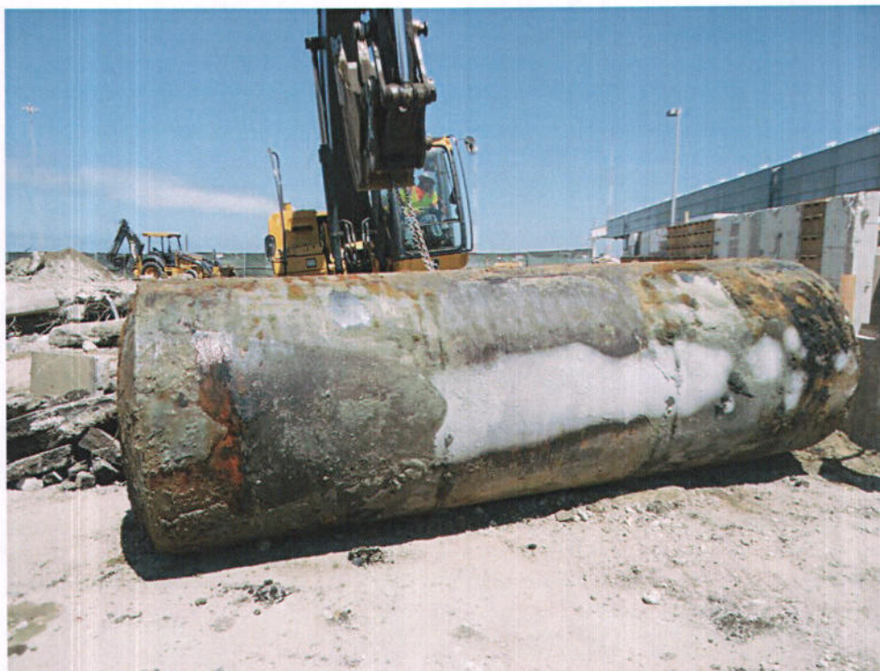
Photo 4 – View looking at UST #1 after it was removed from the ground.
