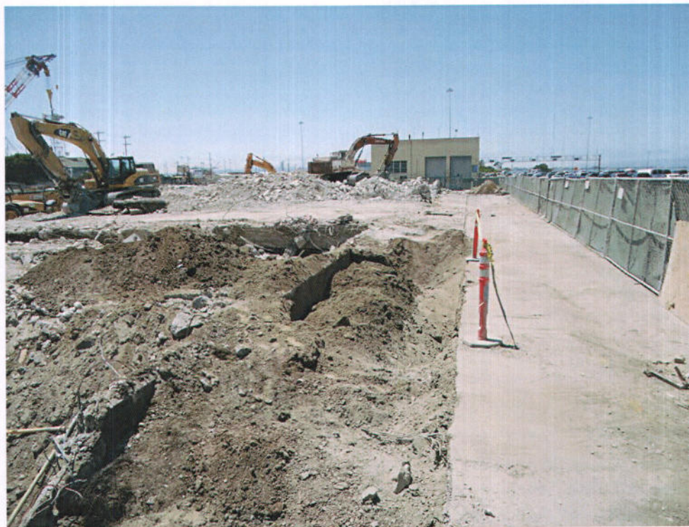
Photo 12 – View looking west at UST #2 after removal and backfill with native soil.
