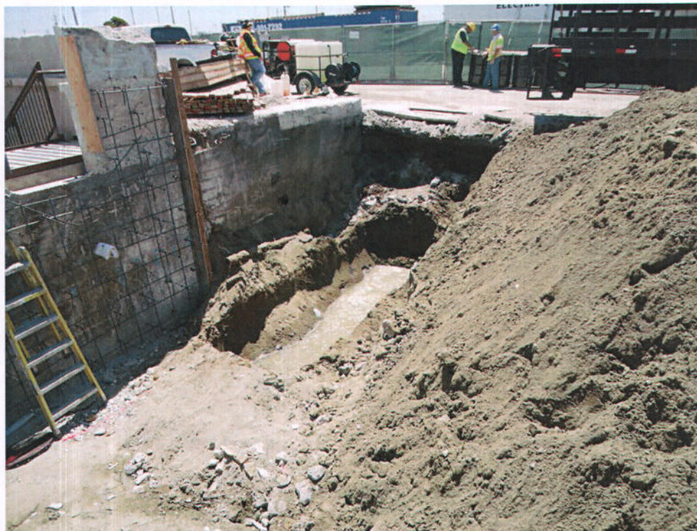
Photo 5 – View looking southeast at groundwater pooled under UST #1.
