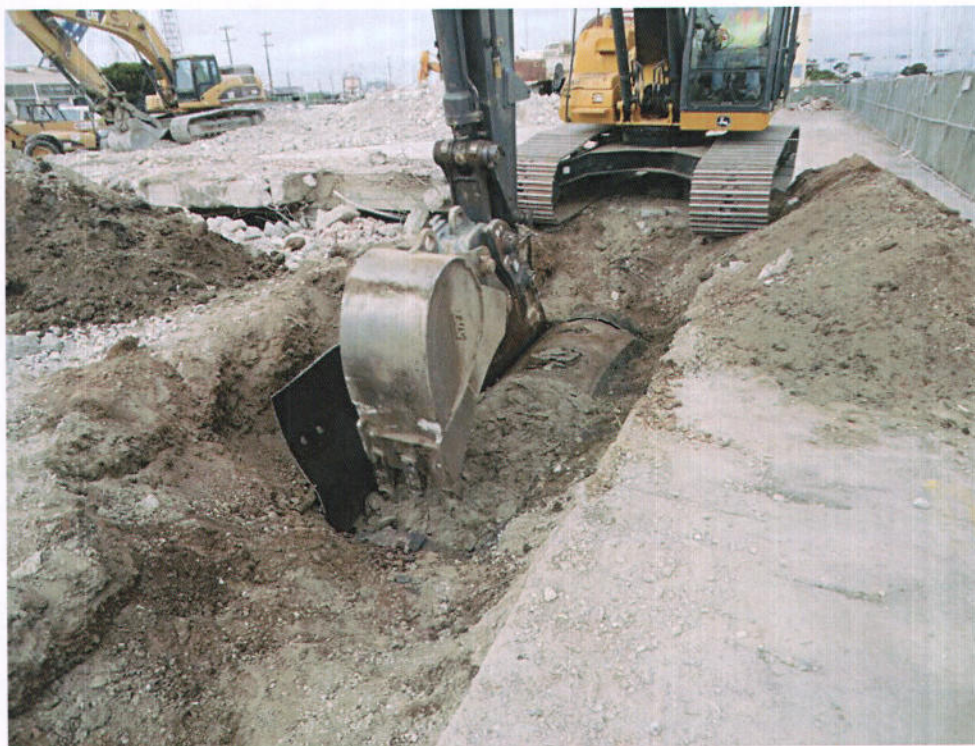
Photo 10 – View looking west at UST #2 while sand slurry is being excavated out of vessel.
