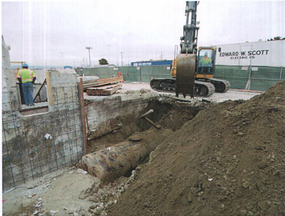
Photo 1 – View looking southeast at UST #1 being unearthed.
