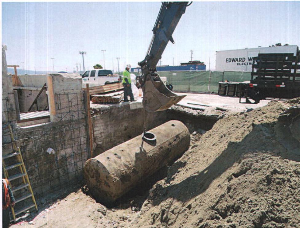
Photo 3 – View looking southeast at UST #1 being removed from ground.
