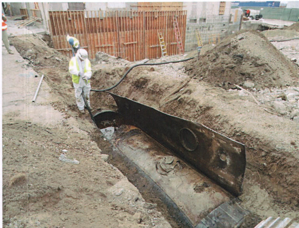
Photo 9 – View looking southeast at UST #2 as diesel #2 is being pumped off surface of sand slurry.
