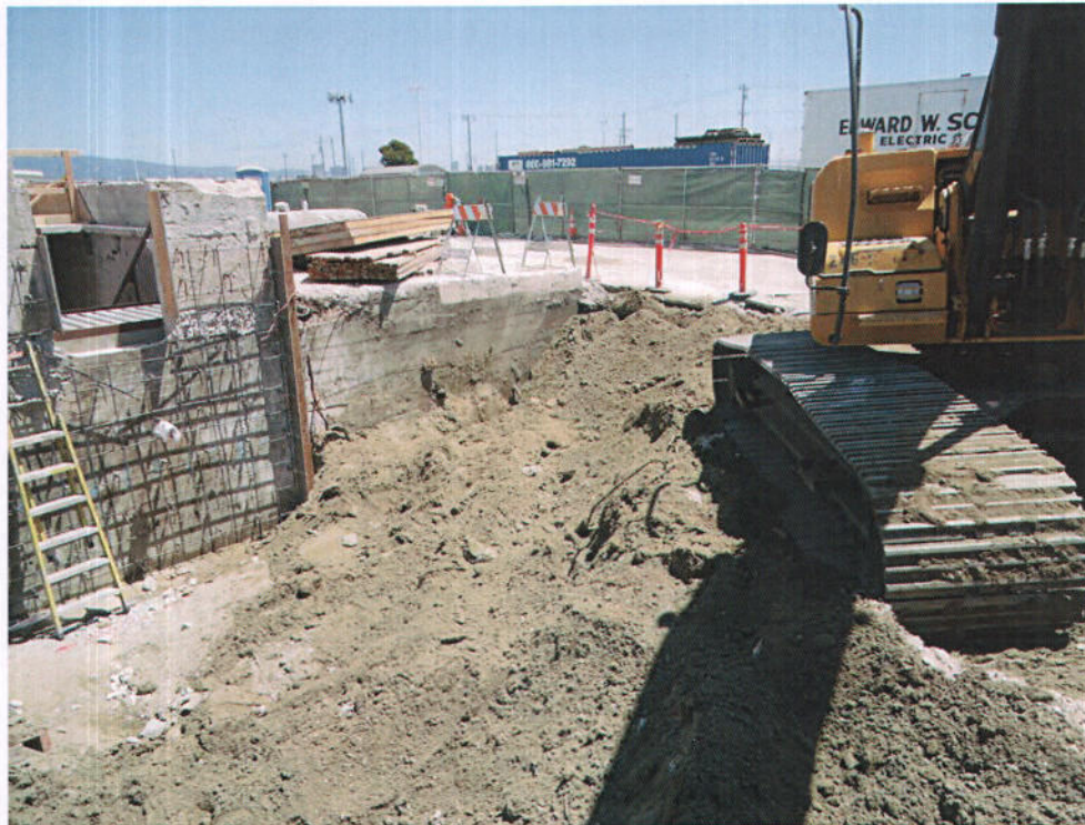
Photo 7 – View looking southeast at UST #1 area after backfilled with native soil.
