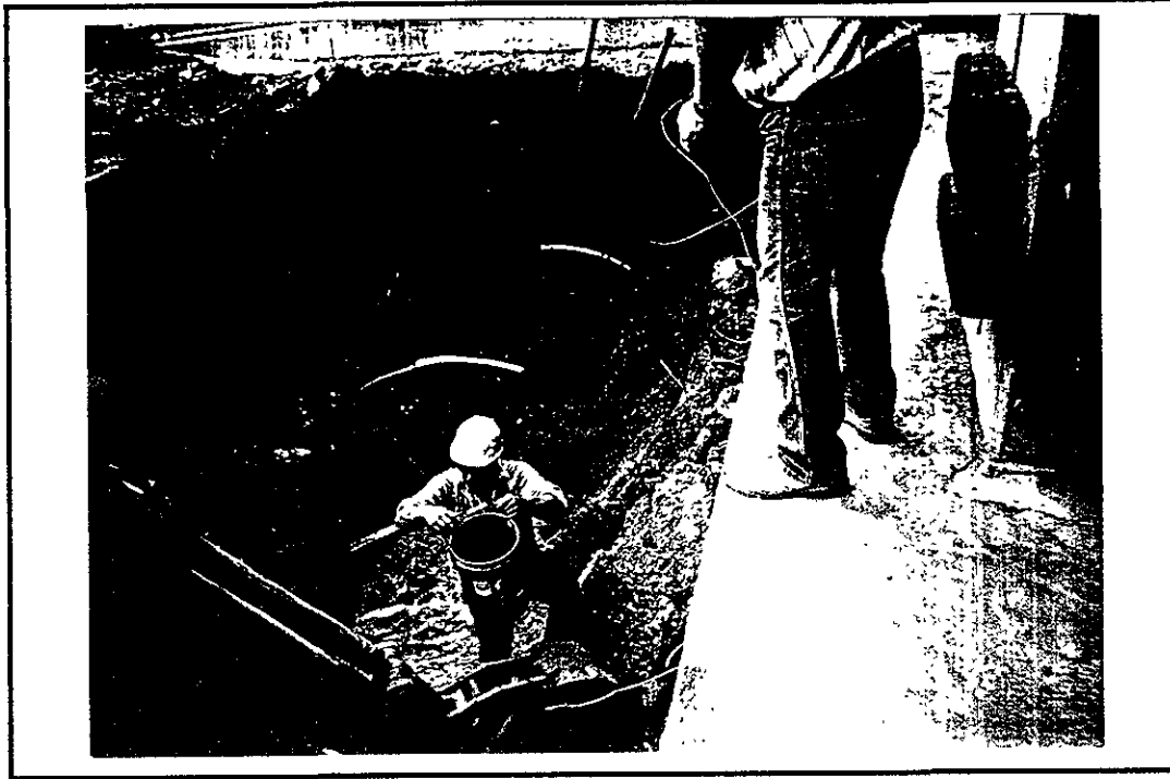
Photo 5: Water sampling from the bottom of the UST excavation.
