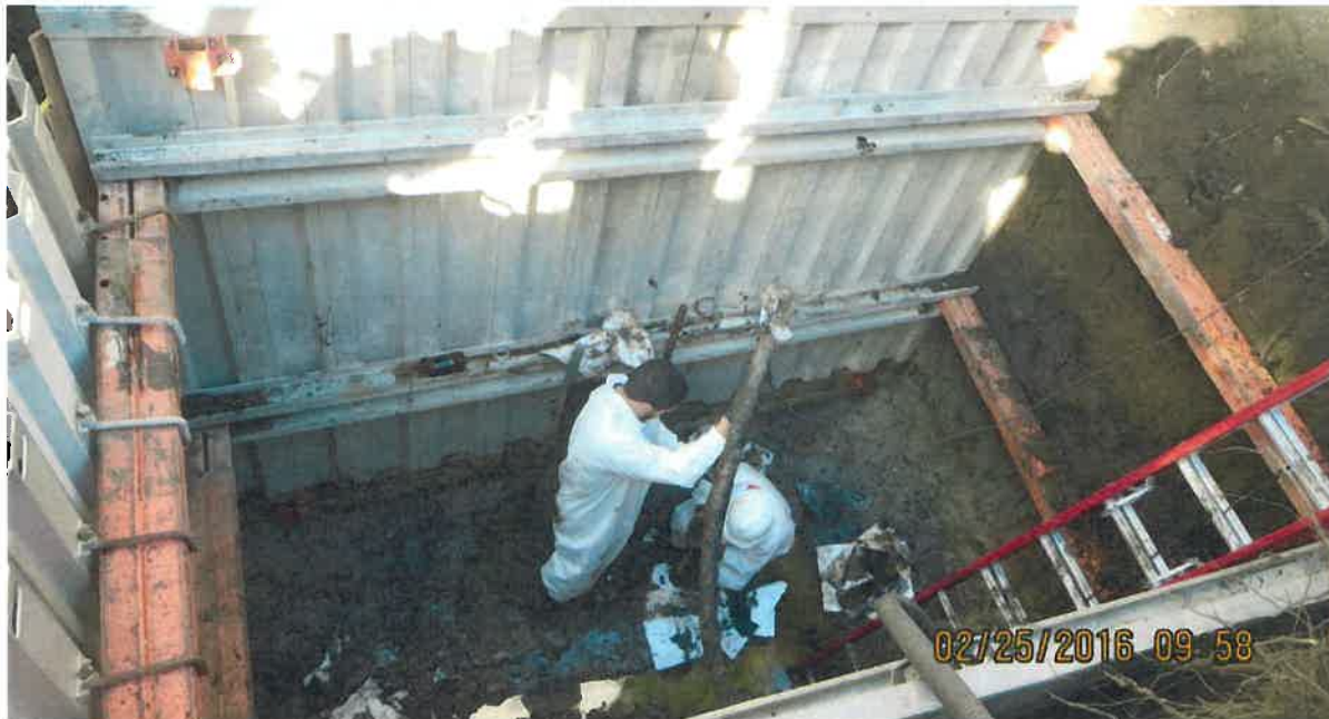
DESCRIPTION: TANK HOLE EXCAVATION – VACUUMING OF RESIDUAL SLUDGE FROM TANK
