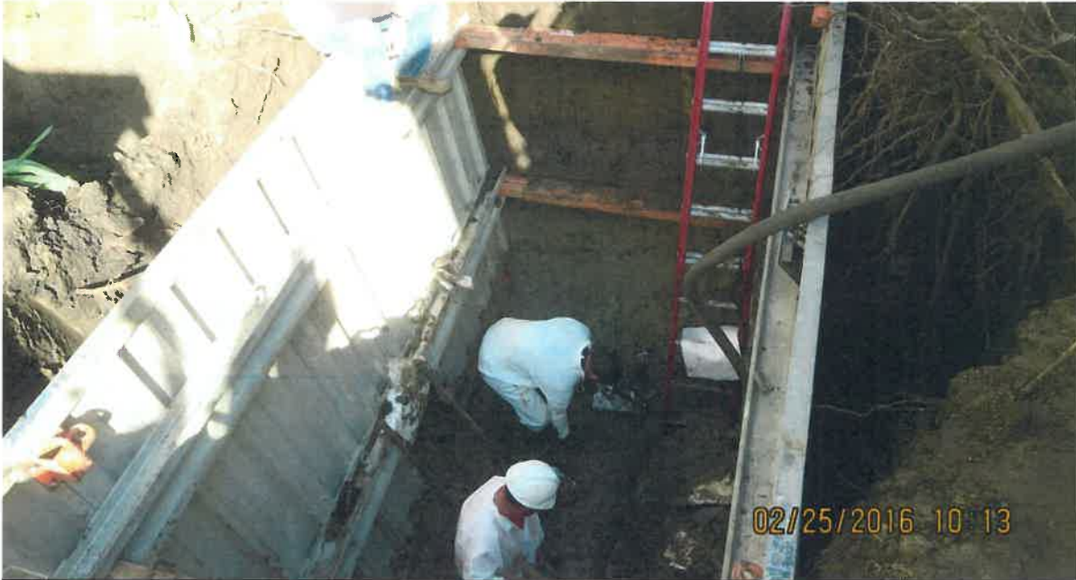
DESCRIPTION: PREPARATION TO COLLECT NORTH WALL SOIL SAMPLE
