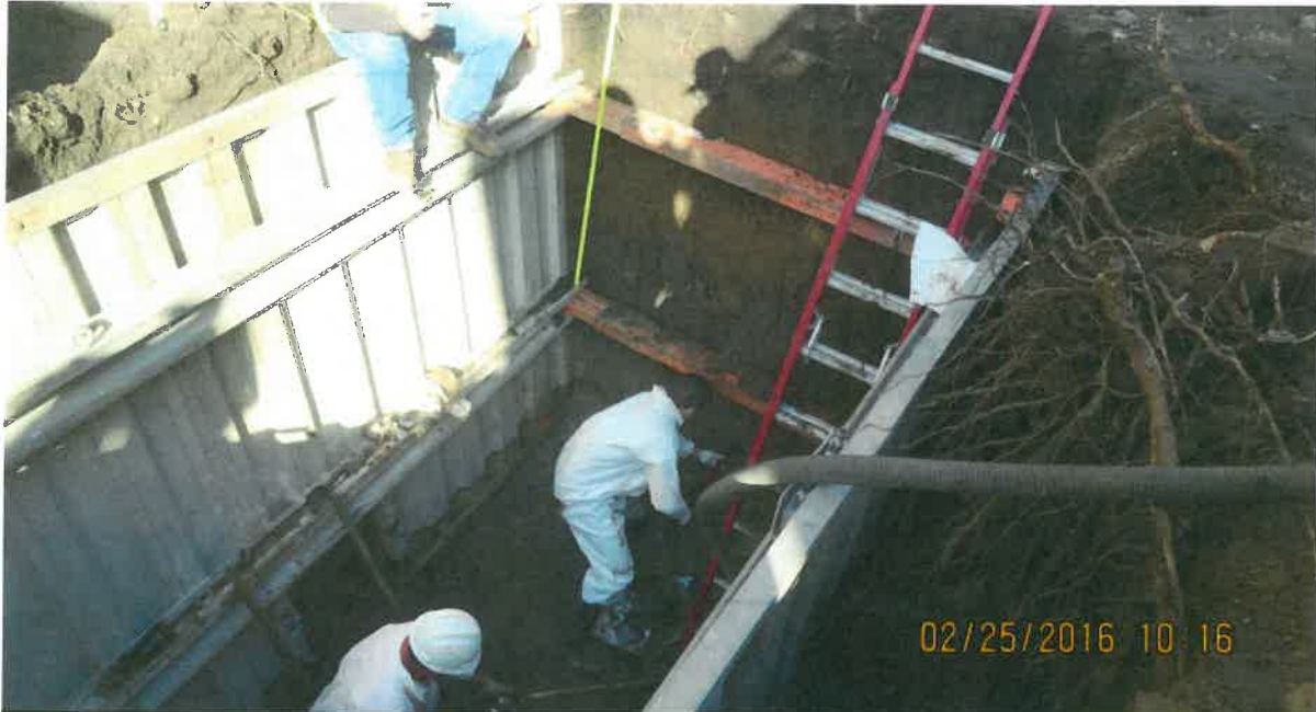
DESCRIPTION: COLLECTING NORTH WALL SOIL SAMPLE
