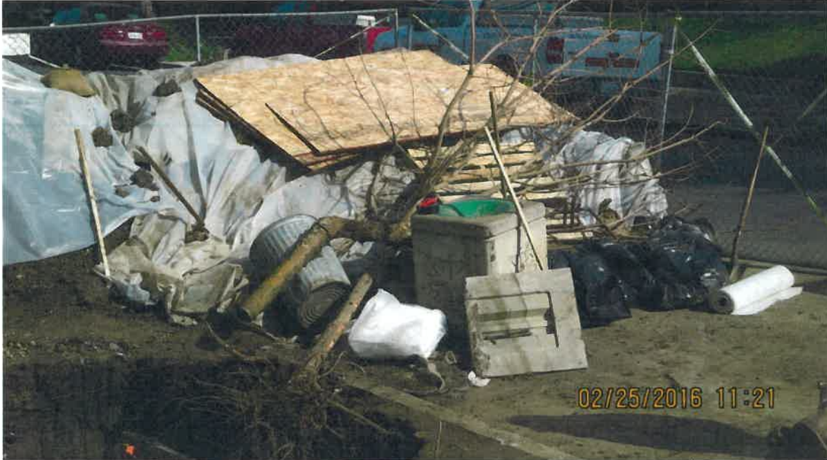
DESCRIPTION: VENT PIPE REMOVED. Photo # 23 of 25
