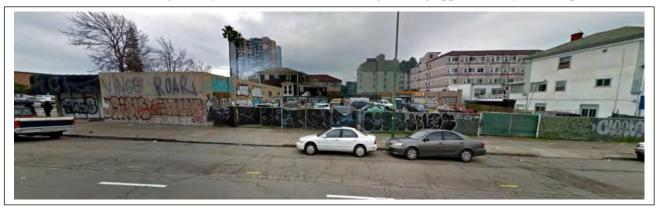
The existing 229 International building was originally constructed in 1951 as an auto service garage. It is one story, rectangular plan, on the west central part of the parcel. It has a vehicle access door at its northeastern corner. Exterior walls are concrete block. The foundation is concrete slab-on-grade. The roof is flat and composition. Its present use is unknown.
