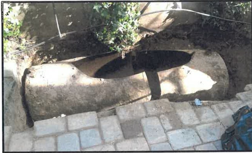
TANK IN EXCAVATION
