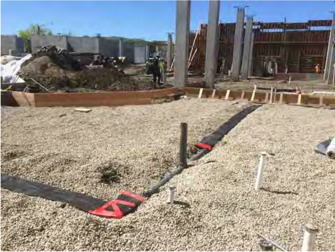
Installed 3rd riser
