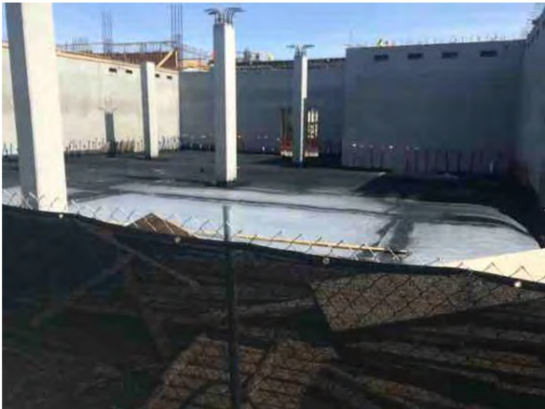
Sprayed out 3/4 of the pad
