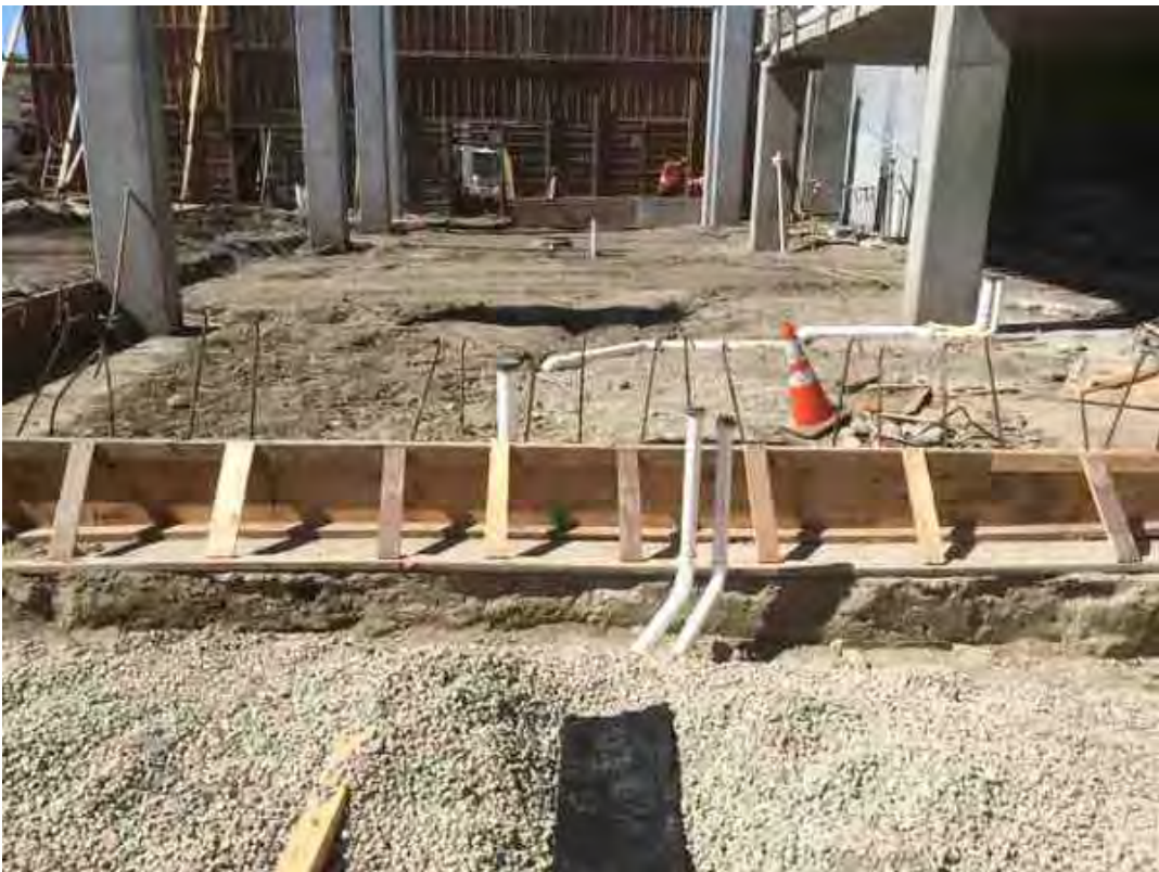
Needs graded and rock
