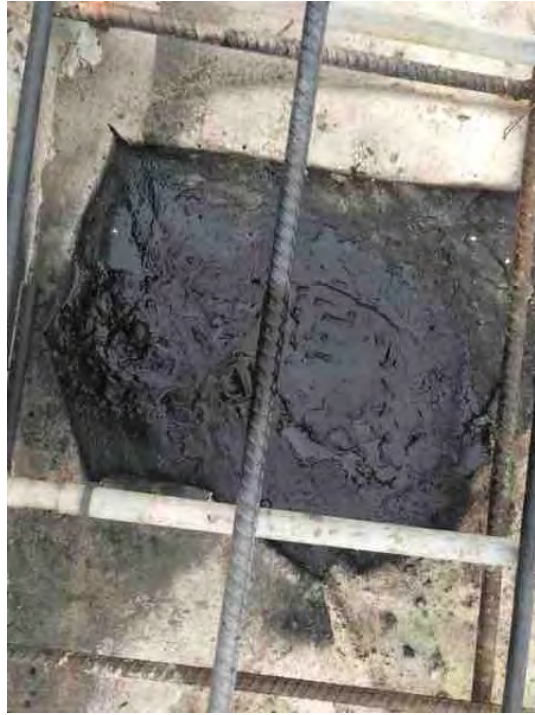
Patched the holes
