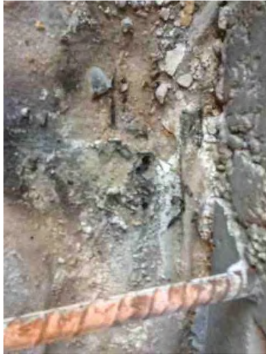
Burn hole in The membrane
