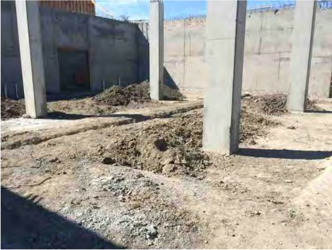
Backfill and grade.
