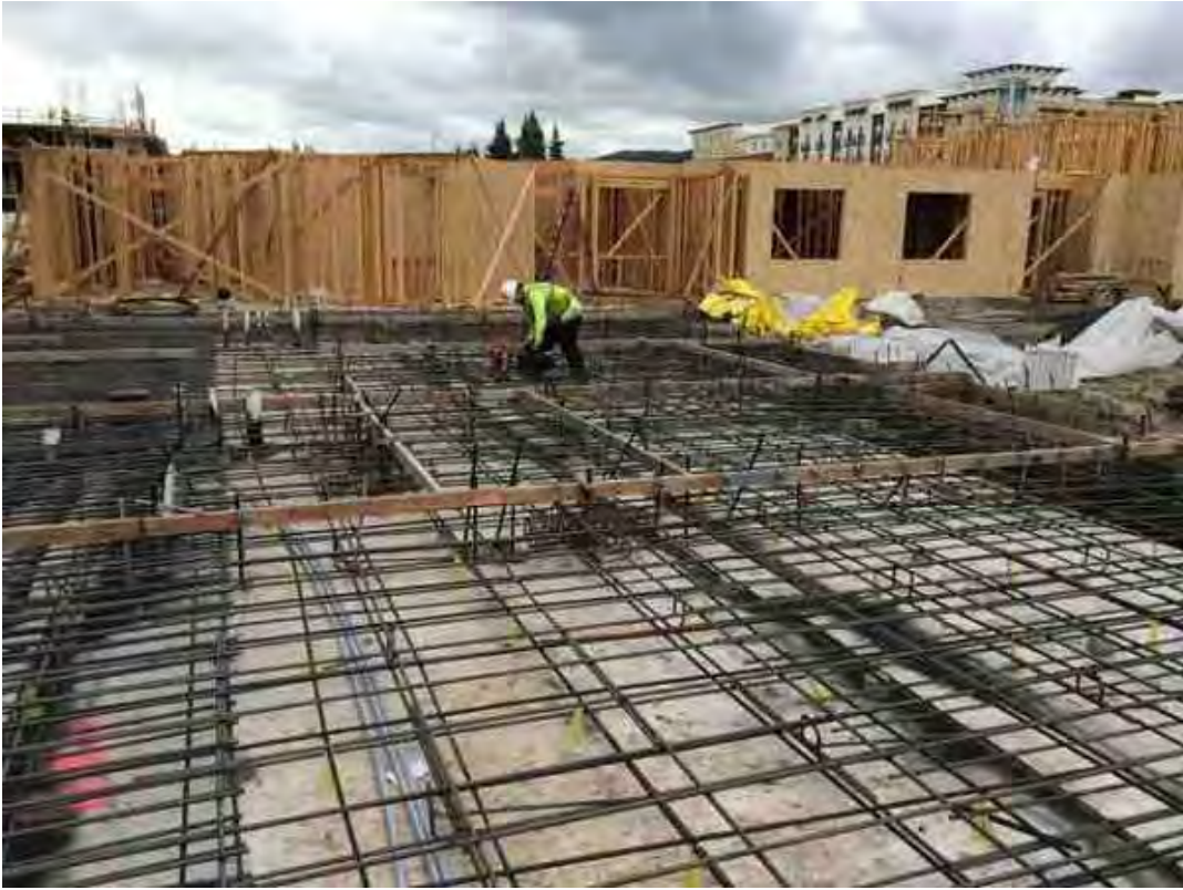
Smoke testing before the inspector gets here to make sure there is no leaks
