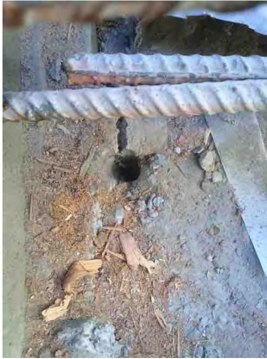
Need to chip concrete and patch big hole
