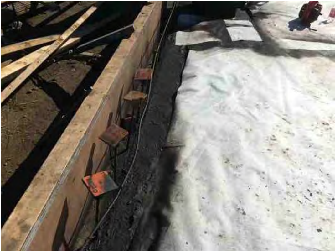
Did 2 repairs on footing on pad F
