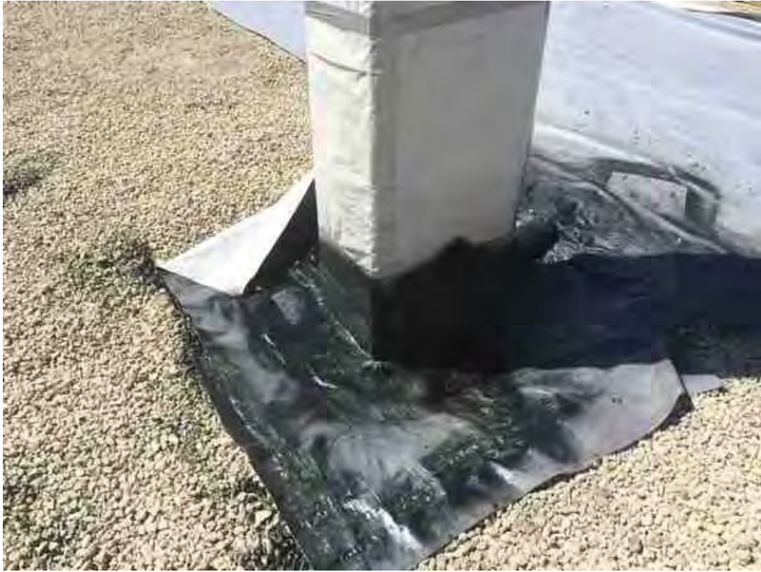
Install target sheets on the columns
