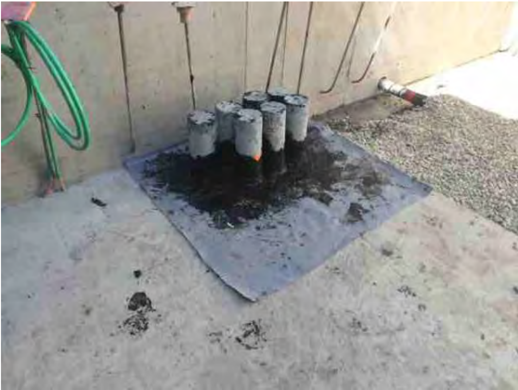
Started penetrations in electric room
