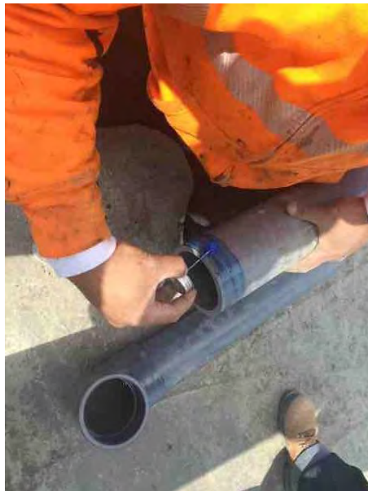
Glued the riser fittings
