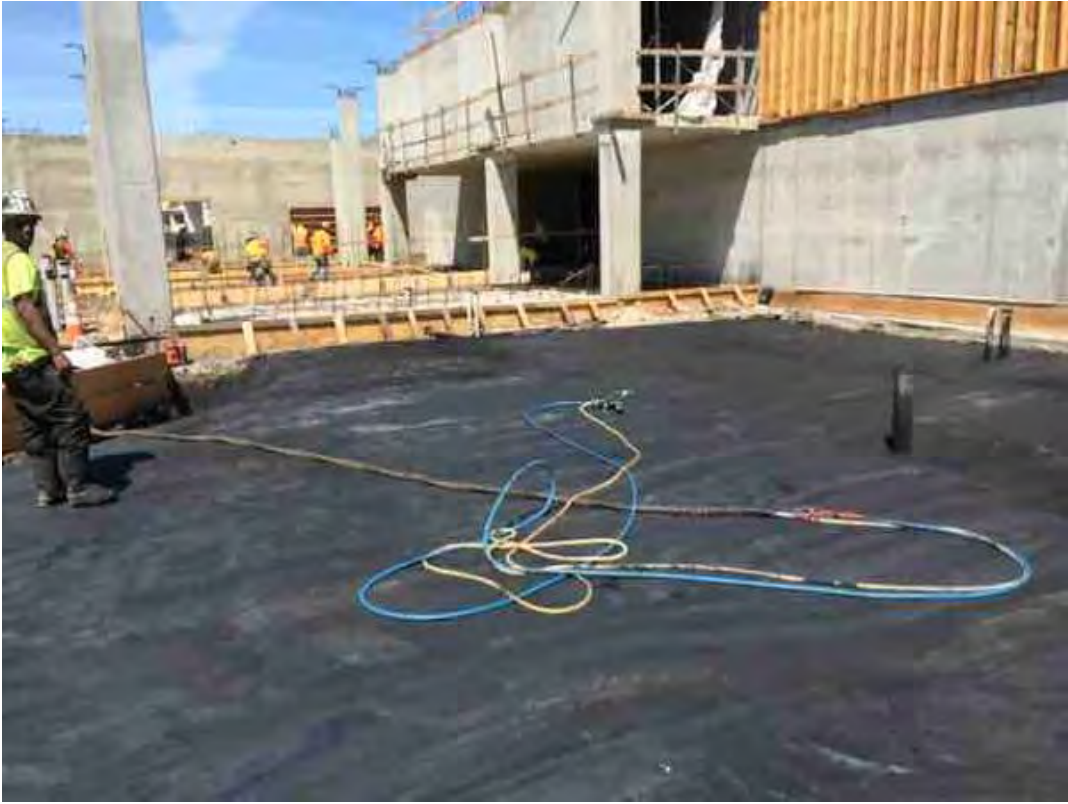
Sprayed out pad
