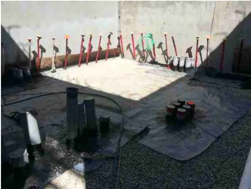
Installed pipe penetrations
