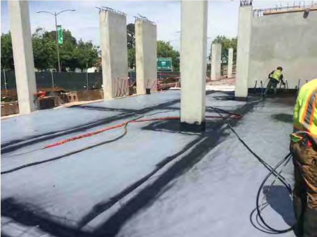
Rolled out base and seeded it
