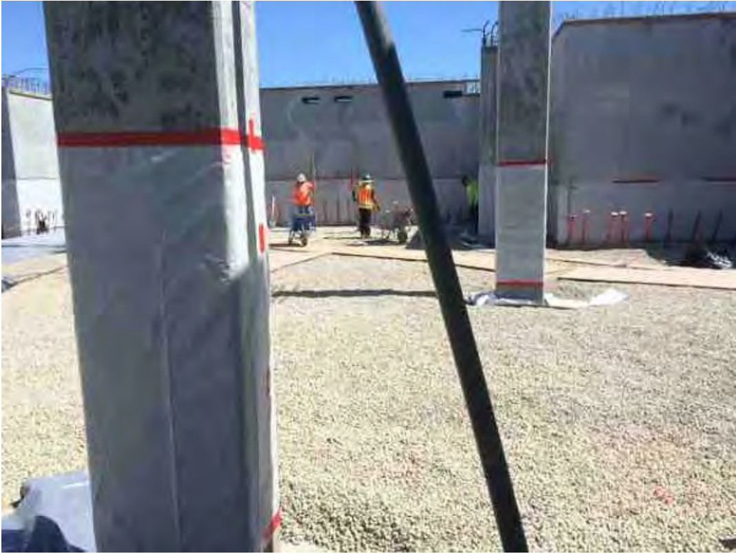
How to remove an inch of rock on the pad
