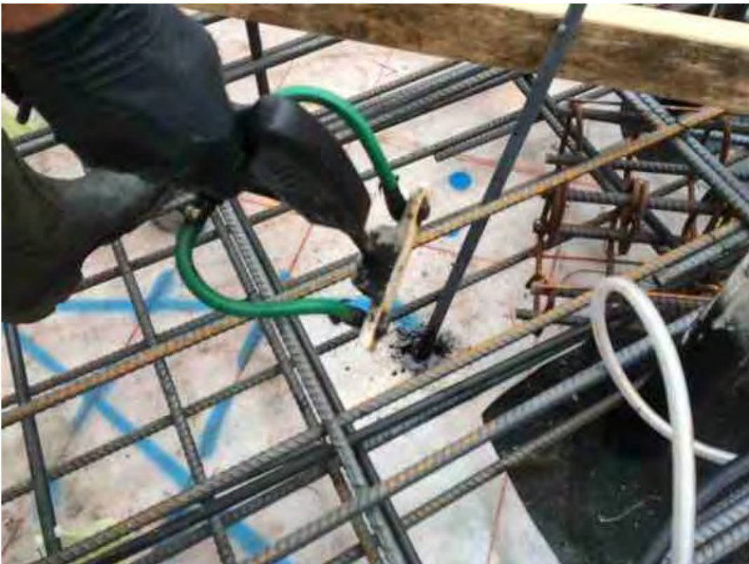
Spraying the vapor stakes carefully
