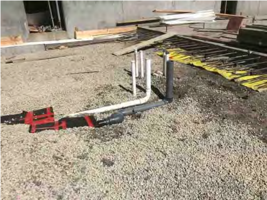
installed 1st riser
