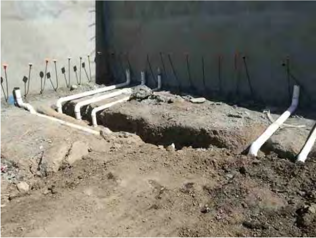
Pad F has a plumbing inspection tomorrow and can be backfilled
