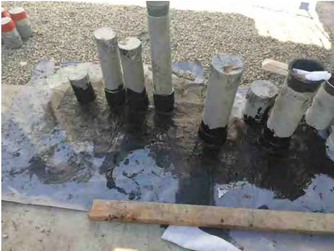
Started penetrations on the electric room
