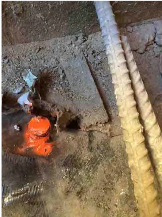
Need to chip concrete and patch big hole
