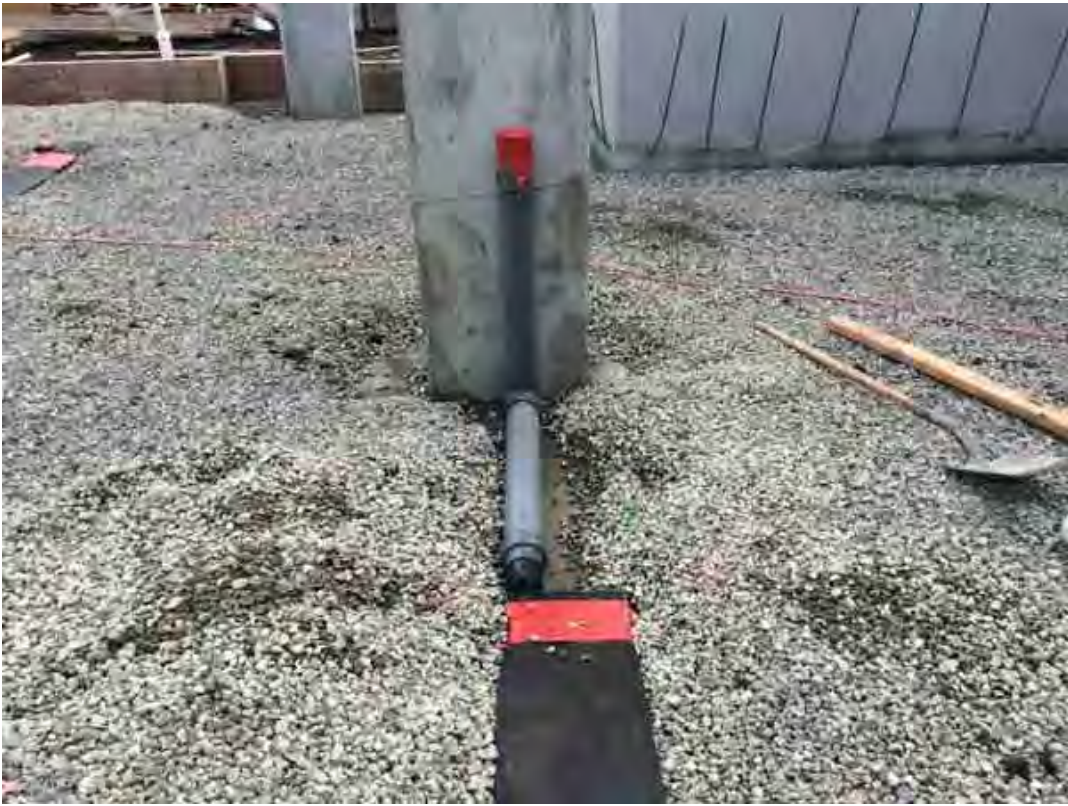
Installed our risers
