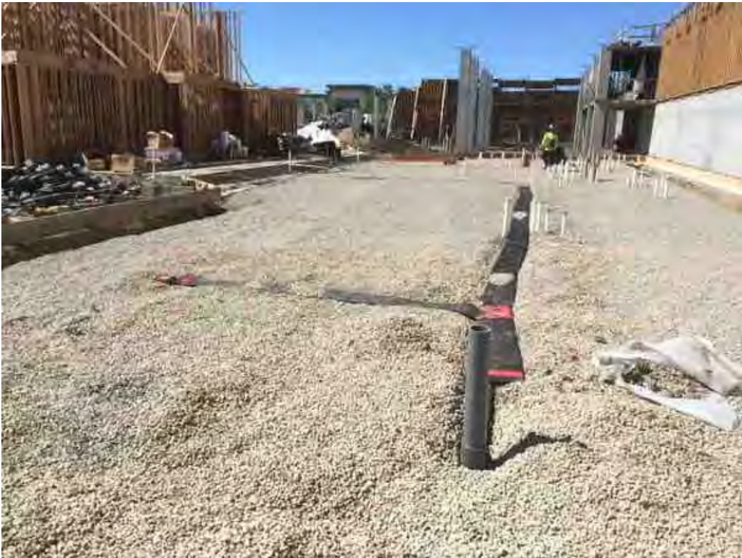
Installed 2nd riser
