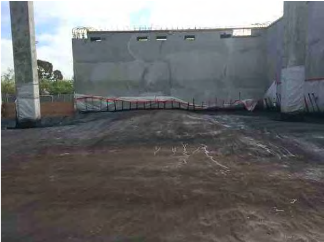
Smoke test on pad E. Lifted the pad
