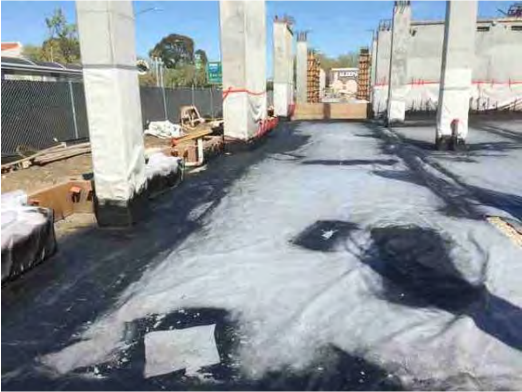
Rolled out and seamed 3,315 sq of material
