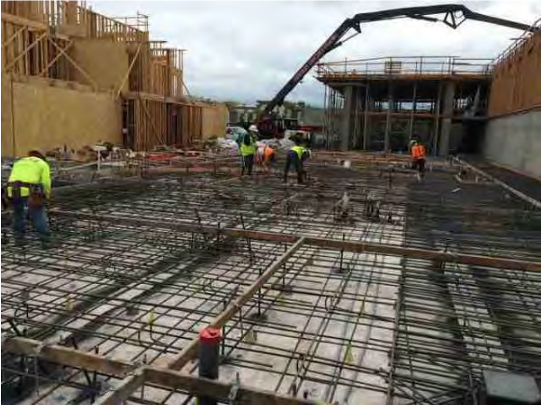
Sealing the vapor steaks
