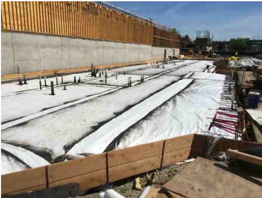
Pre smoked D-2 and installed 7760 sq ft of bond
