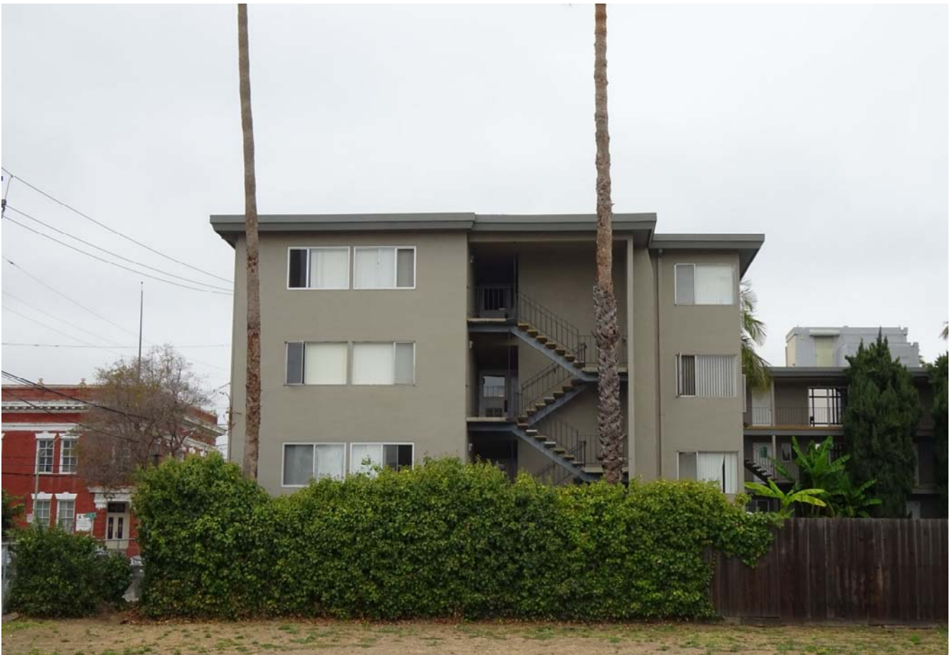
4. View of neighboring property 1720 12th Avenue, located north of the subject property.
