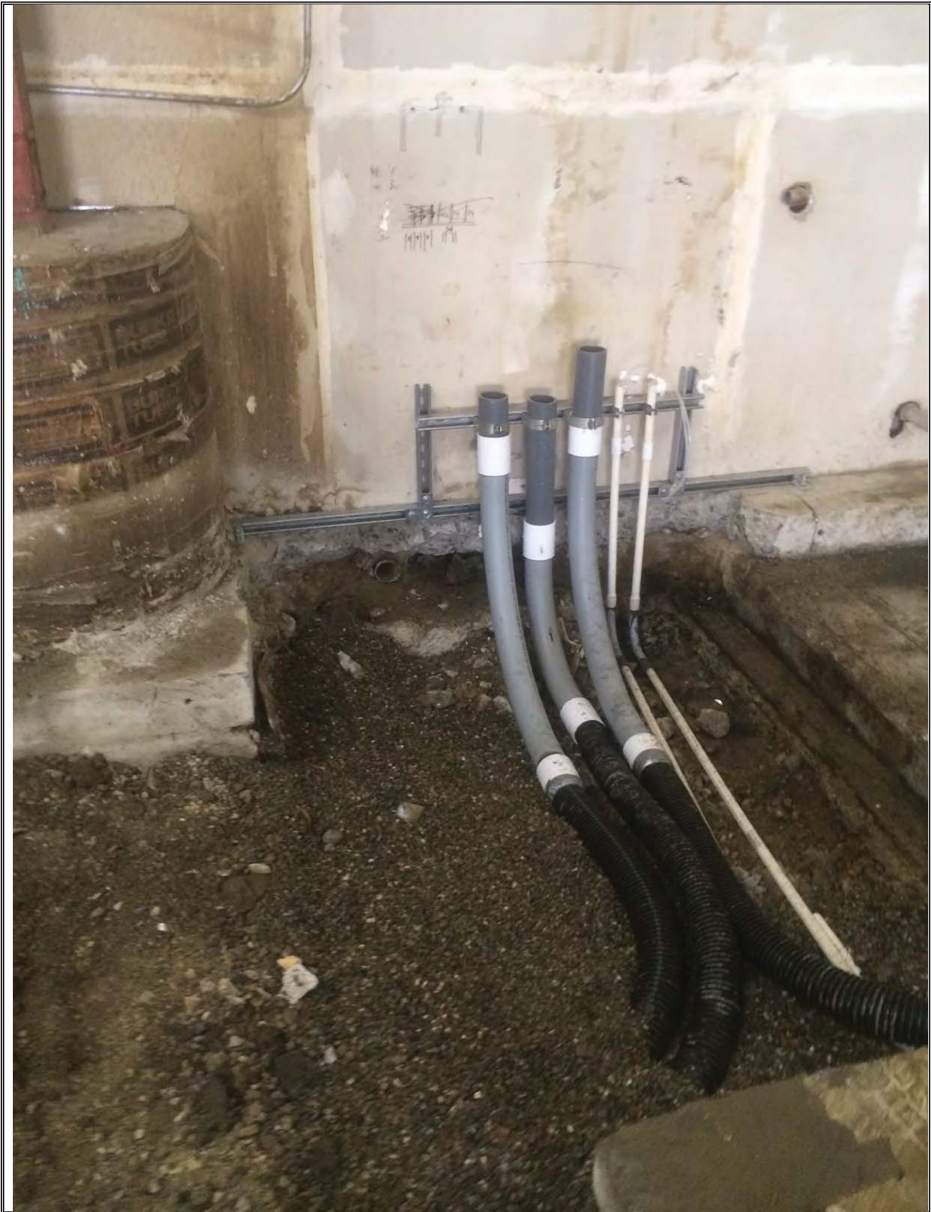
Photo 8 – Manifold with Partial Backfilling
