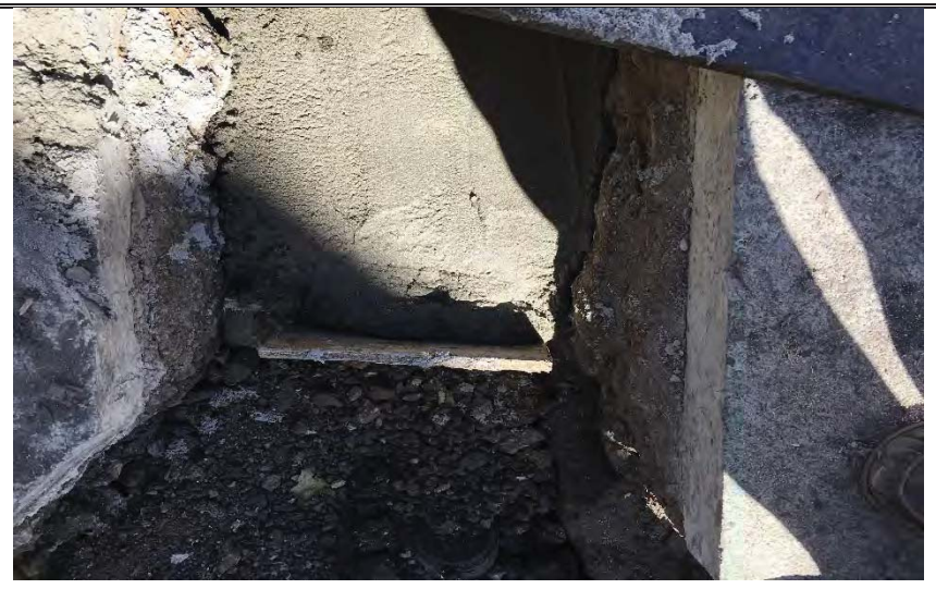
Photo 4. Trench plug in sewer trench south of Building B South.
