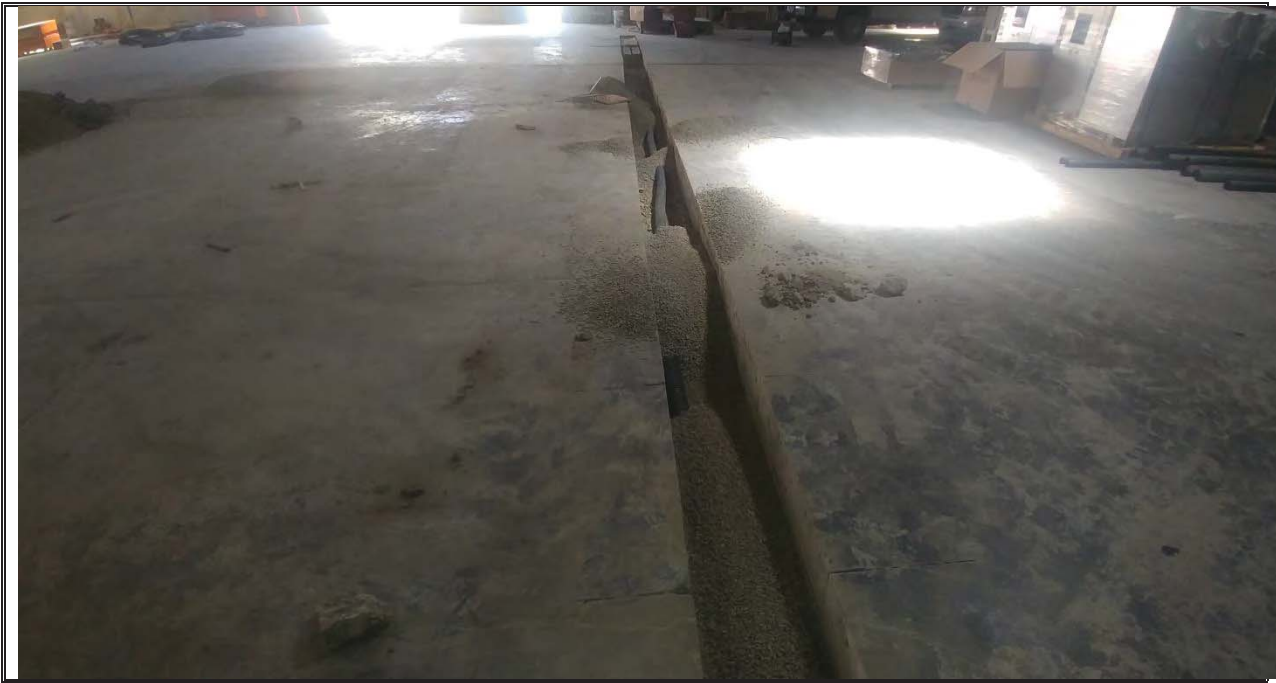
Photo 5 - SSV Piping with Partial Backfill
