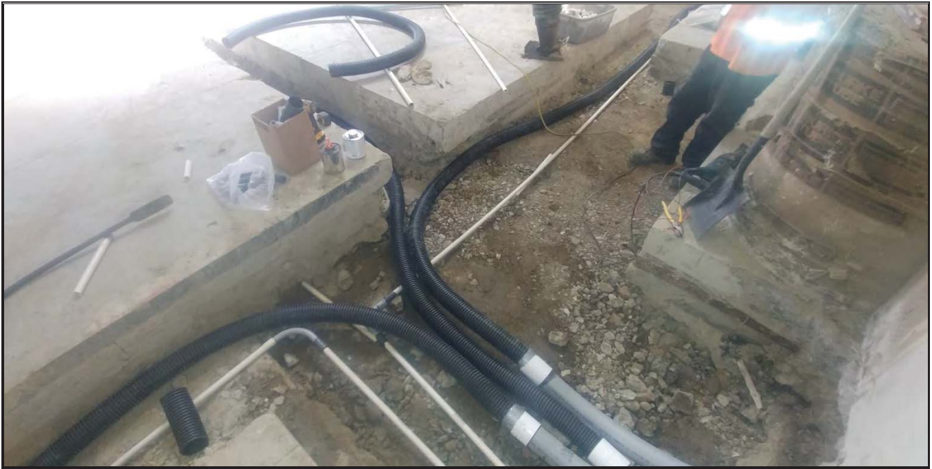
Photo 1 - SSV Piping at Manifold before Backfilling
