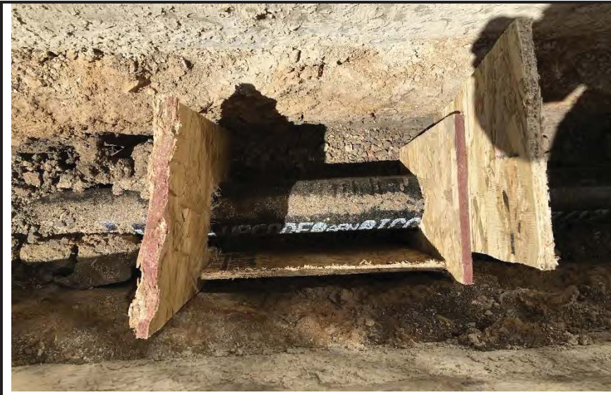
Photo 1. Construction of trench plug in sewer utility trench.
