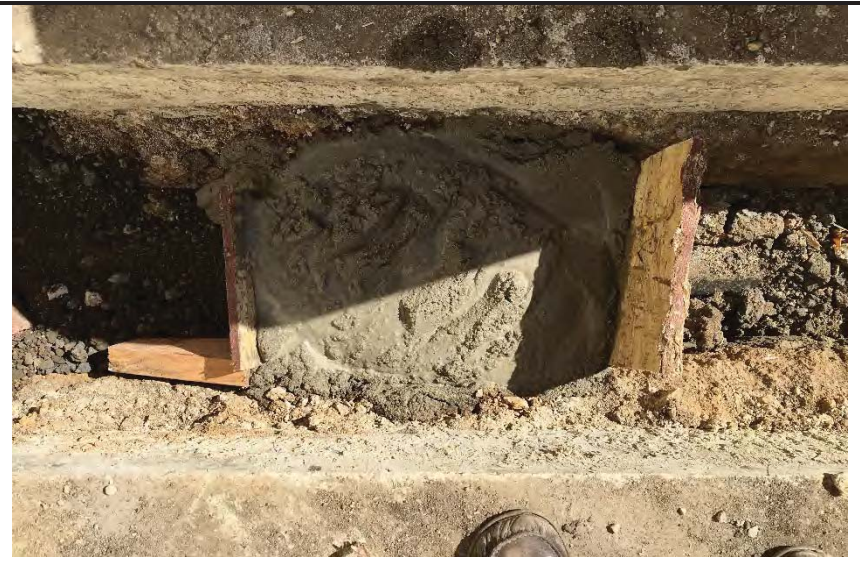
Photo 2. Trench plug in sewer trench south of Building B South.
