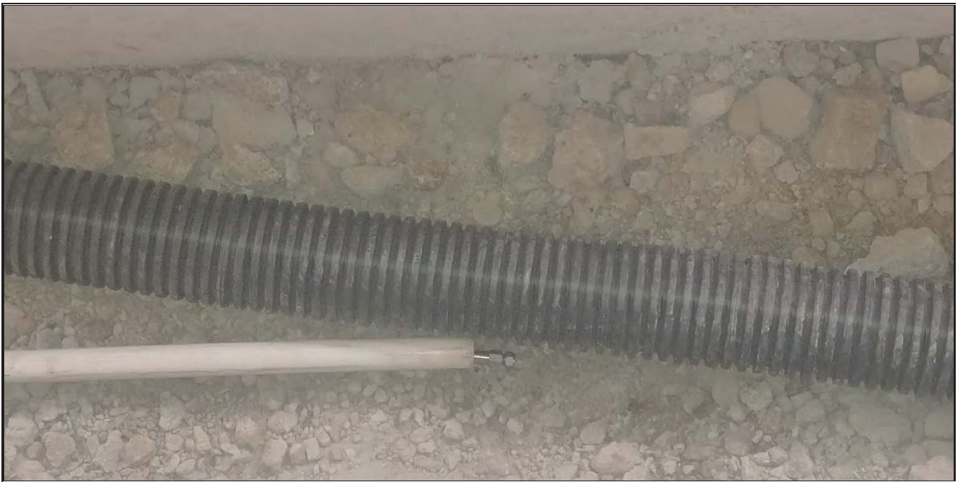
Photo 4 - Sub-slab Probe (Tip and Teflon Tubing) with 3/4" PVC Casing
