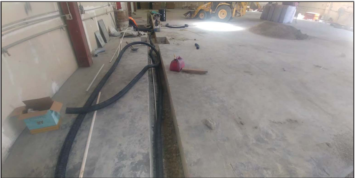
Photo 2 - SSV Piping before Backfilling
