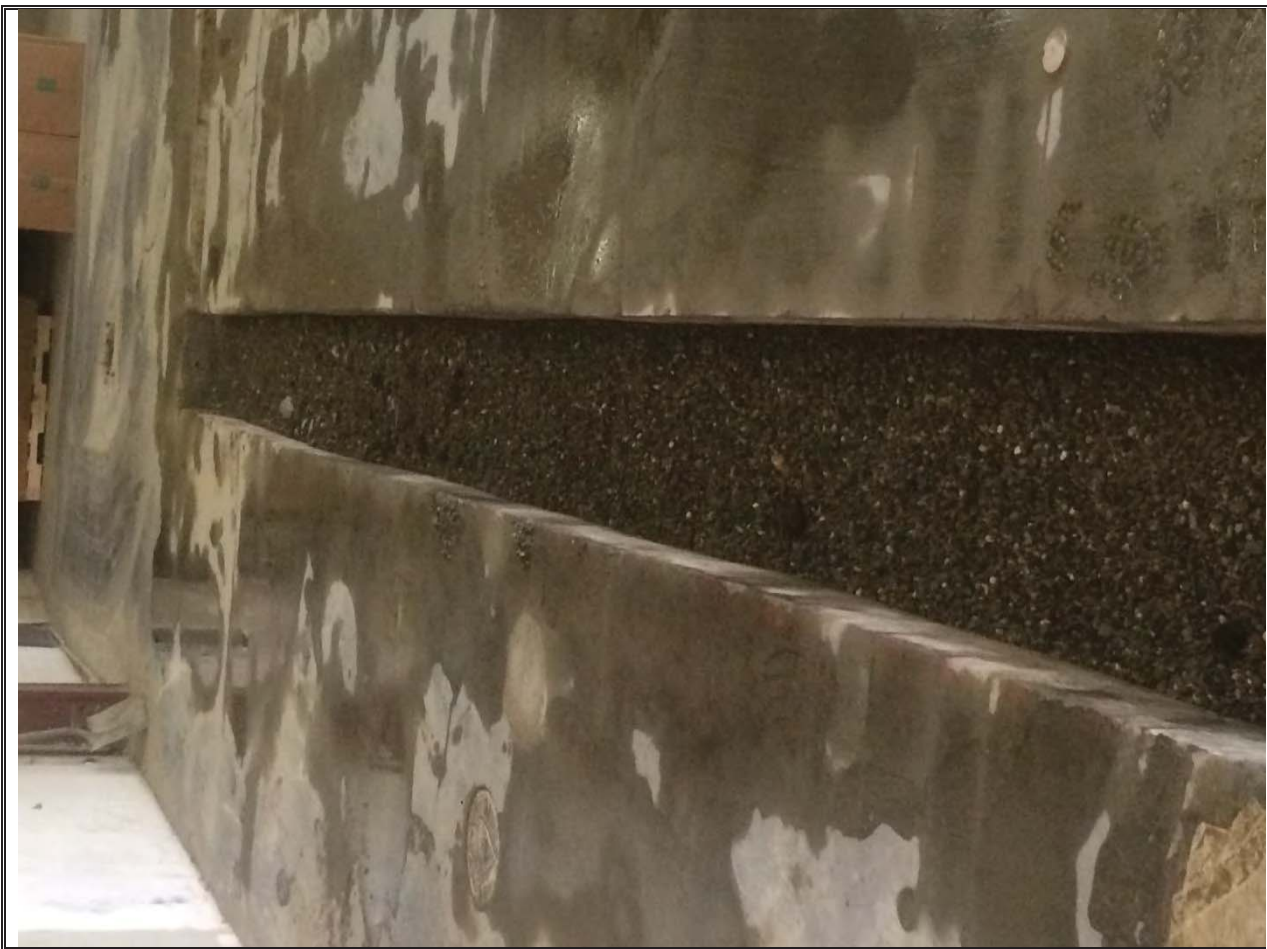
Photo 6 - Trench Backfill Completion
