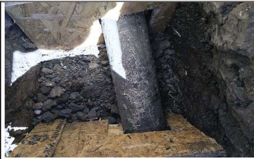
Photo 3. Construction of trench plug in sewer utility trench.
