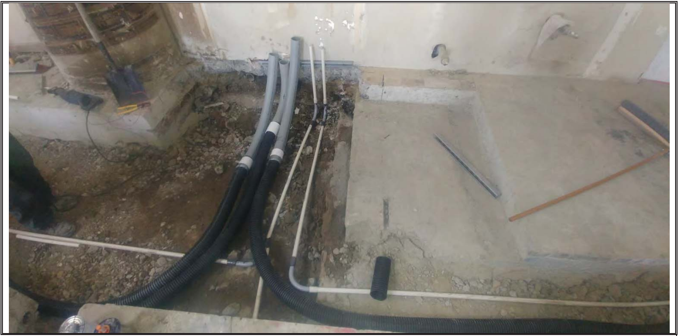
Photo 7-Manifold Stub Ups
