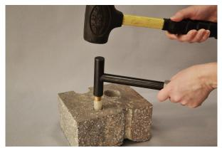
Figure 2. Installing the Vapor Pin<sup>™</sup>.
