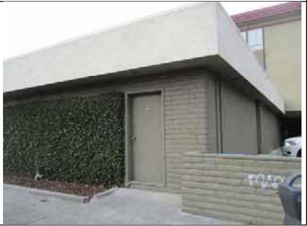
Southeastern elevation of the building viewed from Everett Street.
