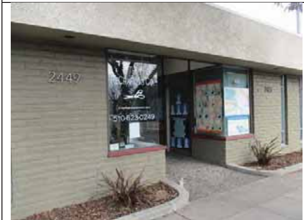
The southwest side of the building.
