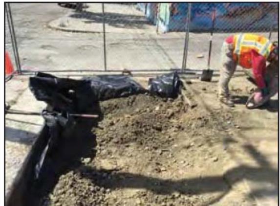
Photograph 24: The fifth UST pit was lined with a 6-MIL polyethylene liner before being temporarily backfilled with the stockpiled soil.
