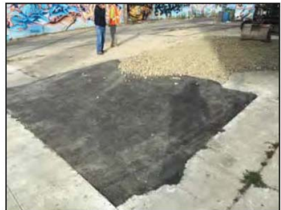
Photograph 18: The area above the third and fourth UST pit was temporarily asphalted over to match the existing grade.
