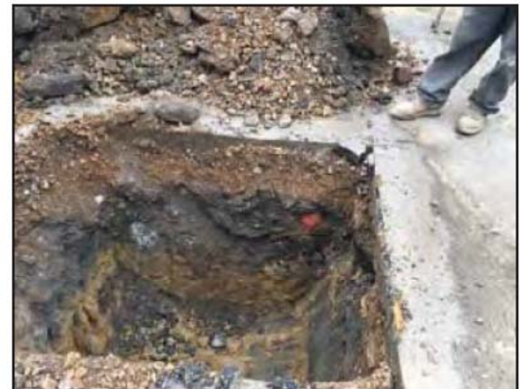
Photograph 30: No green staining was observed in test pit number 3.
