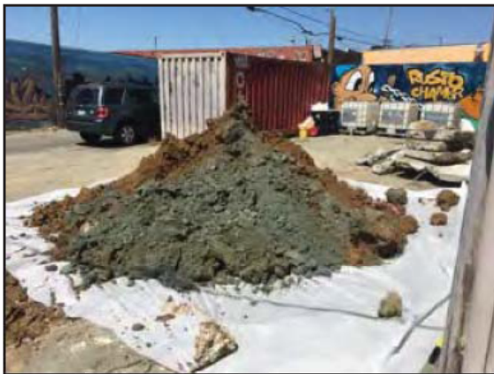
Photograph 3: Excavated soil was stockpiled on a 6-MIL polyethylene liner. Green hydrocarbon staining is visible in the stockpiled soil.
