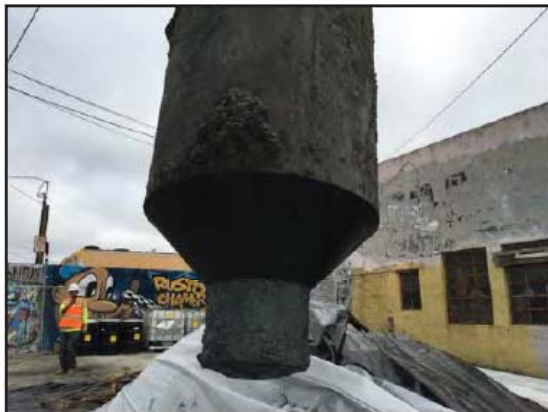
Photograph 23: The fifth UST was found in good condition with no visible holes.
