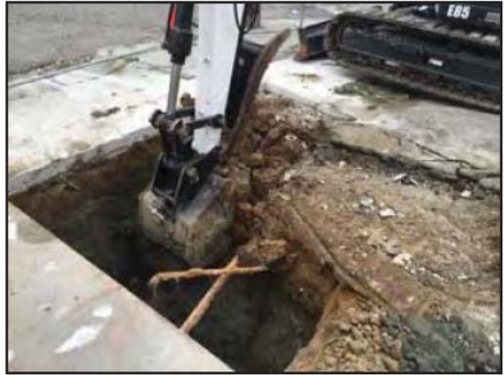
Photograph 8: An excavator was used to expose the fourth UST.
