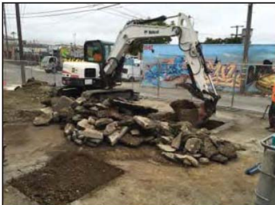
Photograph 29: Test pits were excavated to determine if other USTs existed on site. Test pit number 2 is shown at the bottom left corner and test pit number 3 is shown being excavated on the right.
