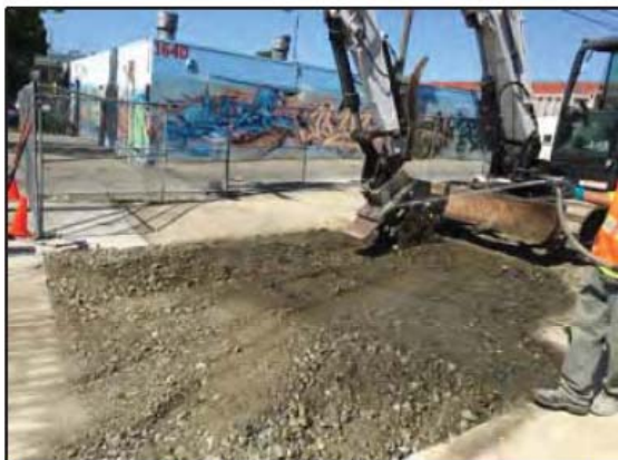
Photograph 17: The backfill was then compacted using a compactor wheel. Water was added to the soil during compaction for dust control.
