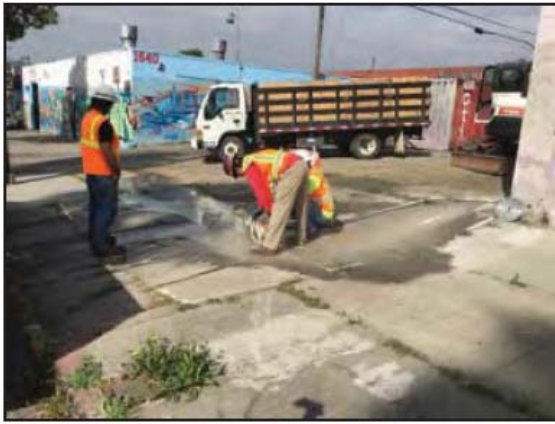
Photograph 1: A saw was used to cut the concrete slab above the third and fourth USTs. The excavation area had previously been cleared for utilities by USA.
