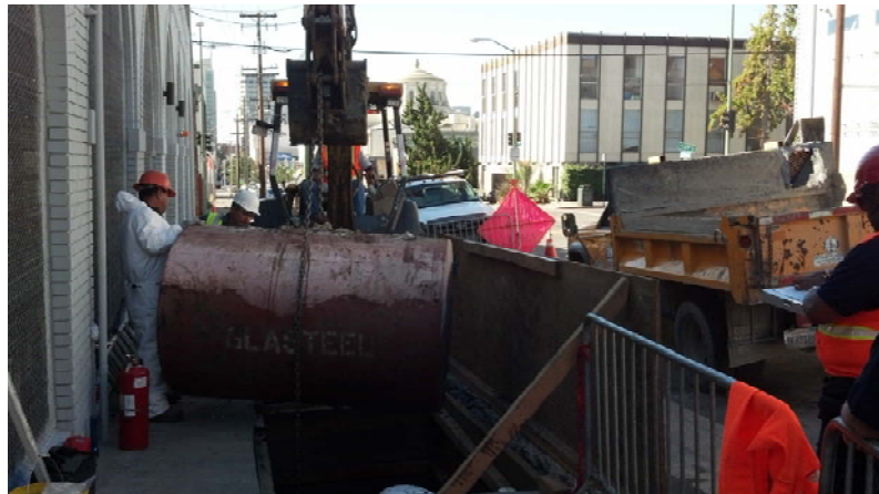
TANK REMOVAL IN PROCESS
