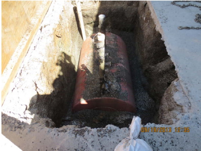
UST READY TO BE REMOVED FROM EXCAVATION
