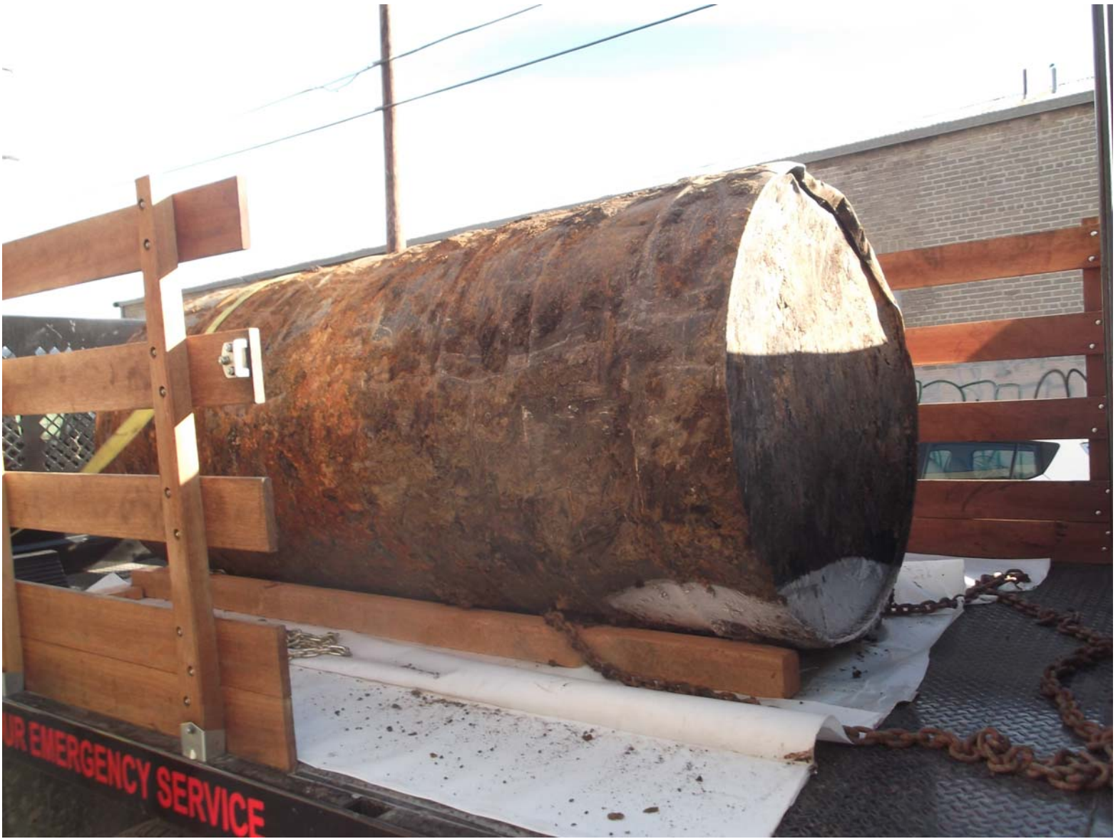
Image #5 UST on truck for transportation.
