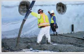
Concrete is placed directly onto the completed Geo-Seal system
