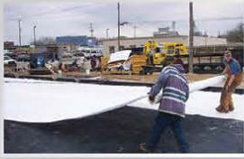
Geo-Seal BOND is applied over the Geo-Seal CORE to provide additional protection
