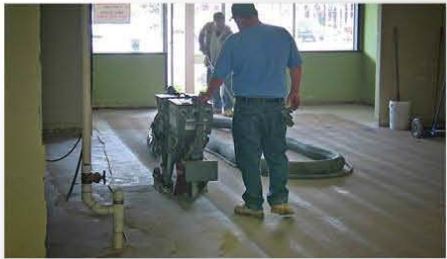
Existing concrete slab is first cleaned and then abraded
