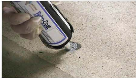
Retro-Coat caulk and fillers are used repair concrete cracks and other imperfections
