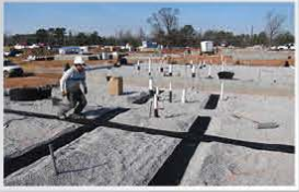
Vapor-Vent should be installed in a permeable subgrade to maximize vapor collection ability
