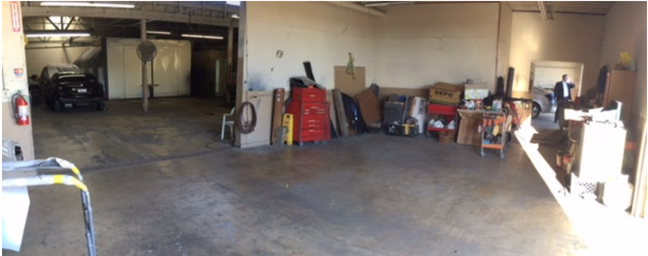
Photo 3: Subject Site (Facing Northwest) One-Story Commercial Garage Building (East Warehouse Area of A&C Auto Body & Frame Unit A)
