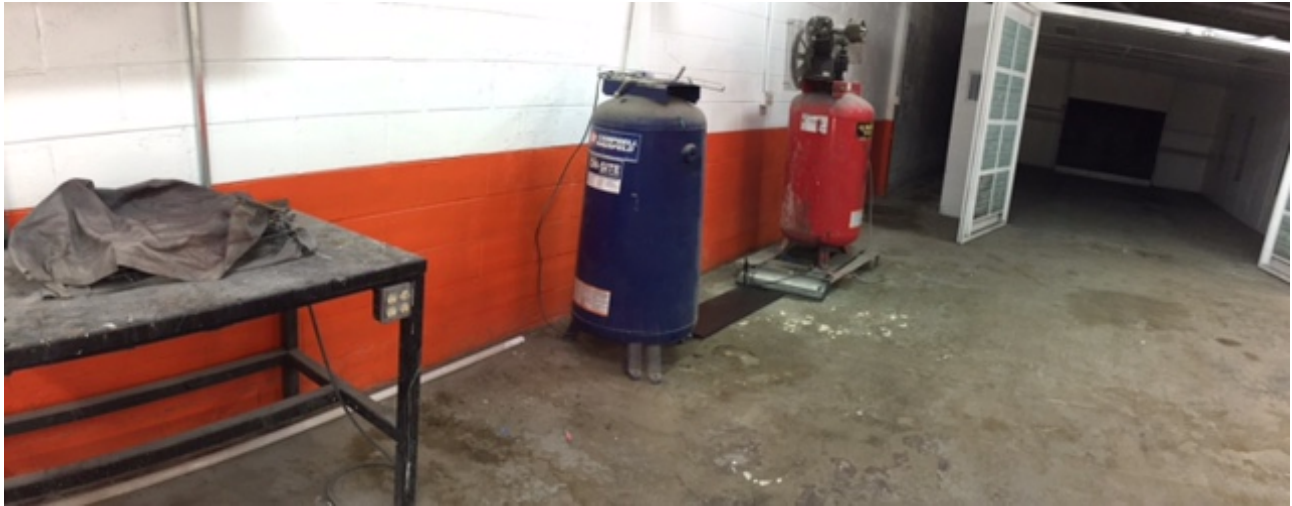
Photo 16: Subject Site (Facing Northwest) One-Story Commercial Garage Building (Paint Booth and Air Compressors in Vacant Retail Unit E)
