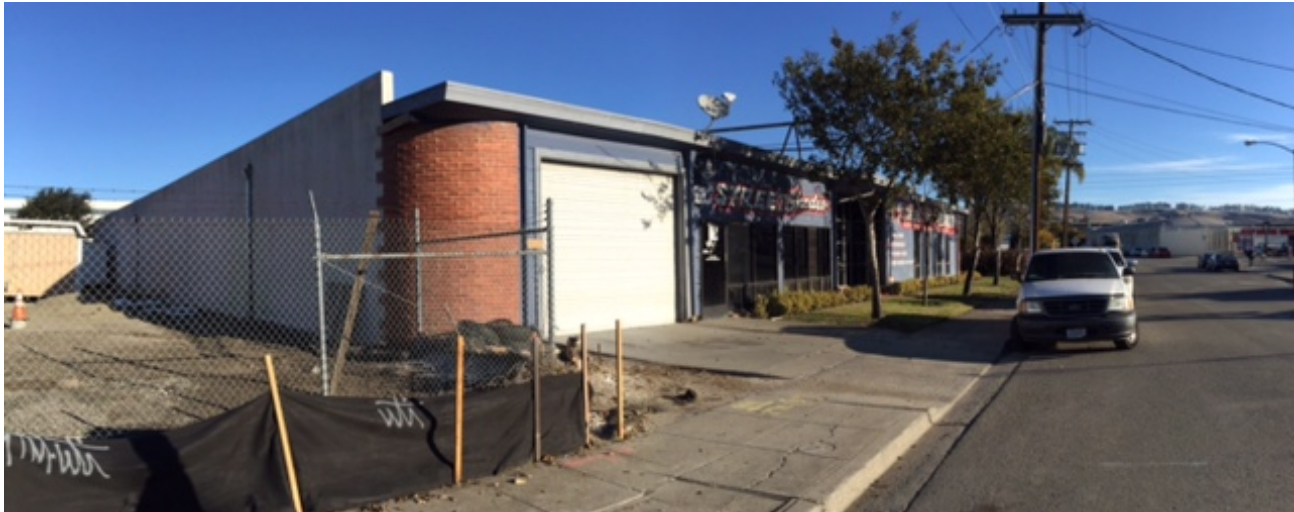
Photo 2: Subject Site (Facing Northeast) One-Story Commercial Garage Building and Associated Paved and Landscaped Areas at the Northwest Corner of 139th Avenue and Washington Avenue
